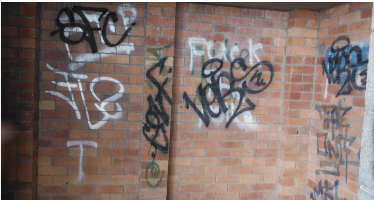
Beneath the stairs of neighbouring building, view from car park
