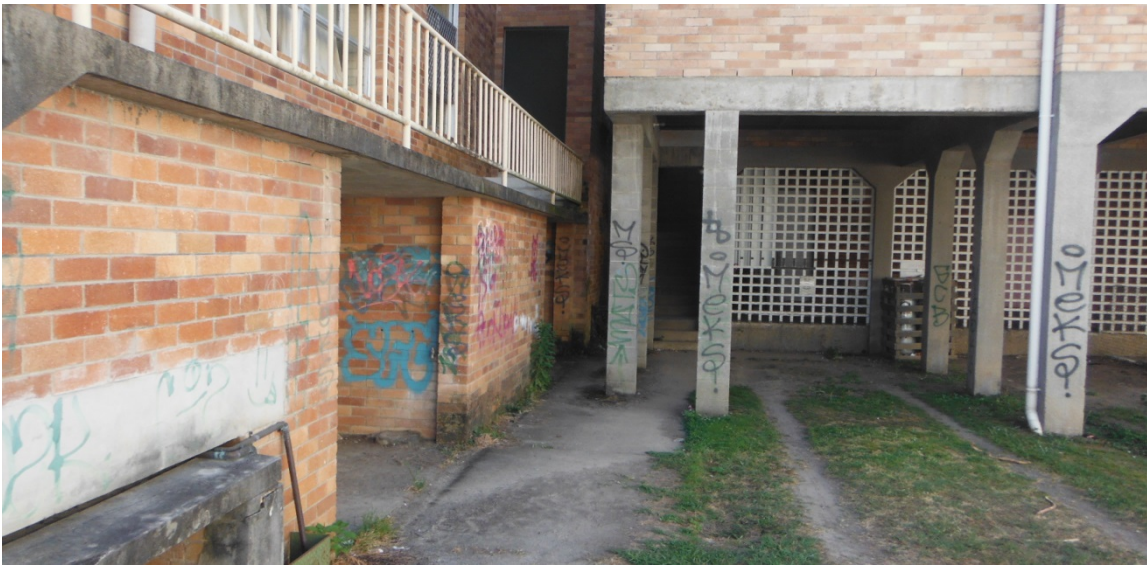
Rear of CWA building from car park
