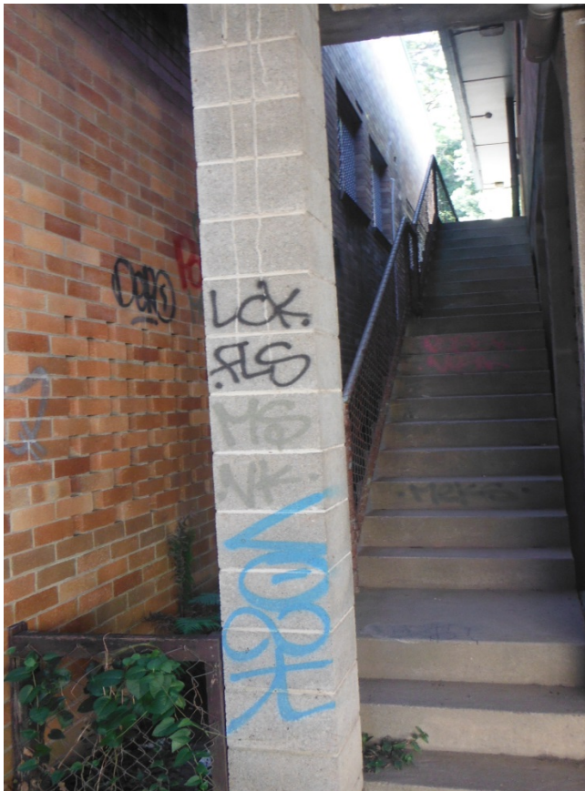
Looking up the stairs from the car park
