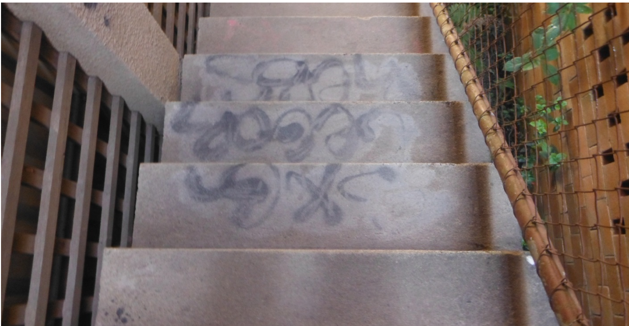
Looking down the stairs, going down to the rear car park
