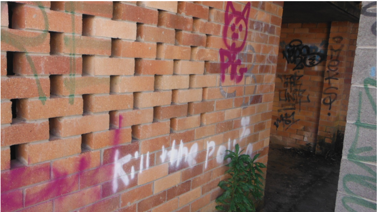
Beneath the stairs of neighbouring building, view from car park
