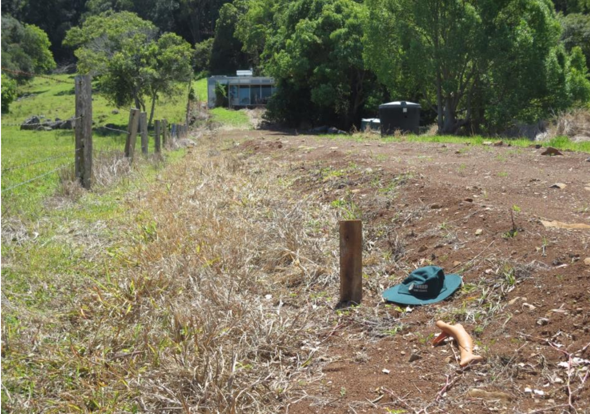
Figure 14: Fill of access to dwelling off River Road
