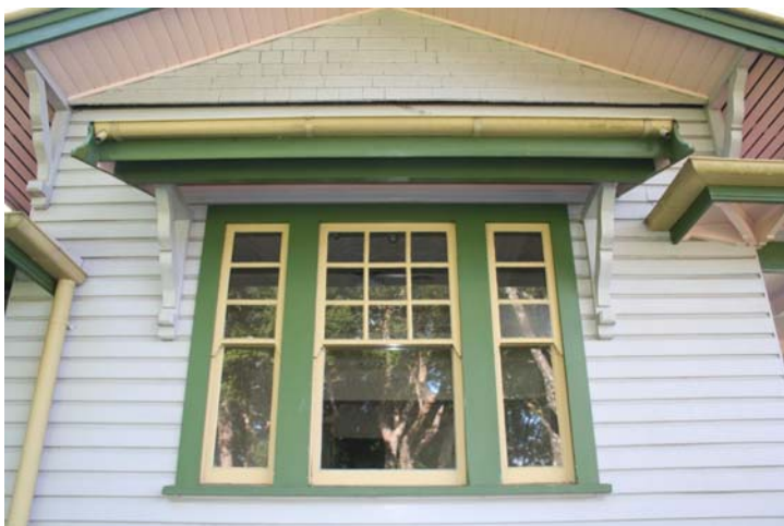
Photograph 33 Original fabric and details – exceptional significance
