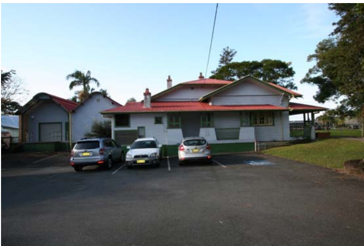
Photograph 66 The complete North Elevation and car park
