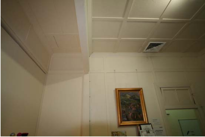
Photograph 106 Room layout altered and bulkhead remains
