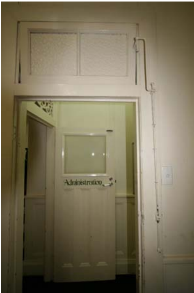
Photograph 104 Original door and toplight with hardware
