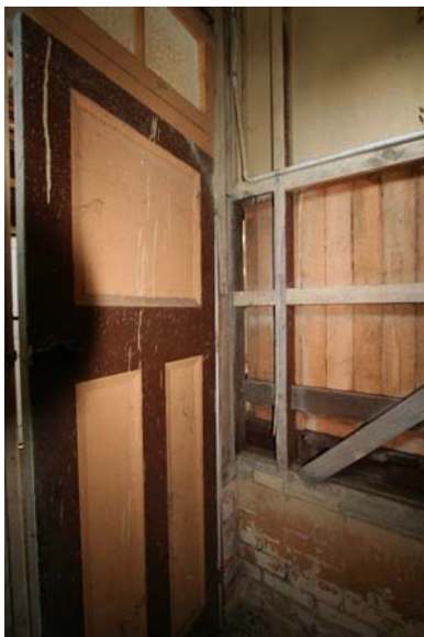
Photograph 12 Original store – former laundry – Exceptional significance
