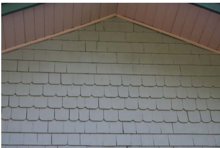
Photograph 36 Original fabric and details – Exceptional significance
