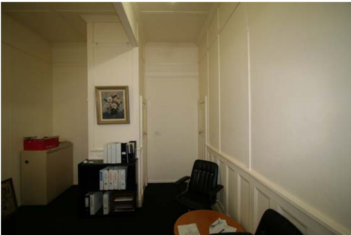
Photograph 119 Exceptional built in cupboard
