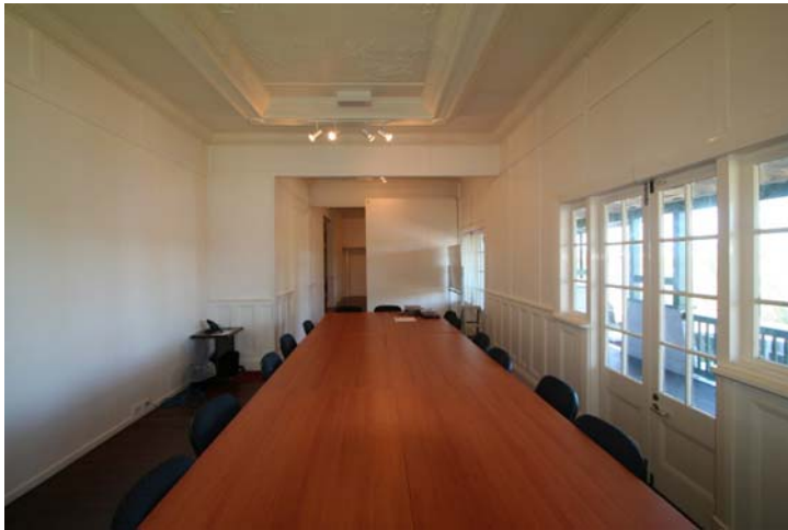
Photograph 5 Modified side walls – moderate level of significance
