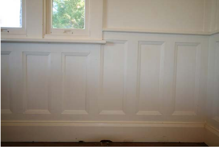
Photograph 149 Note paint removal from rare cedar joinery
