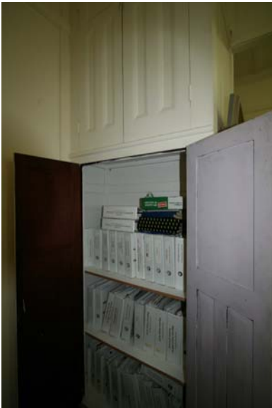
Photograph 110 Exceptional built in cupboard
