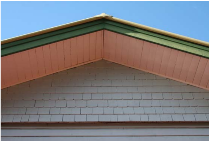
Photograph 38 Original fabric and details – Exceptional significance
