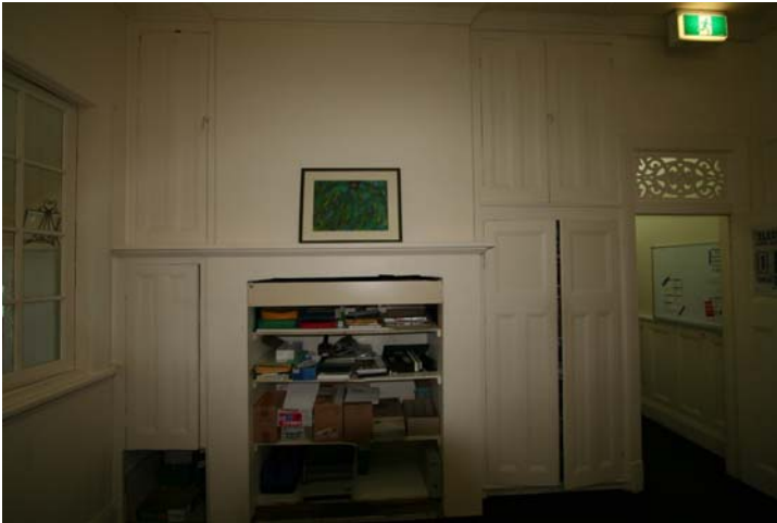
Photograph 98 The kitchen stove area and Exceptional built in cupboard
