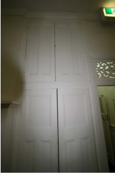
Photograph 97 Exceptional built in cupboard
