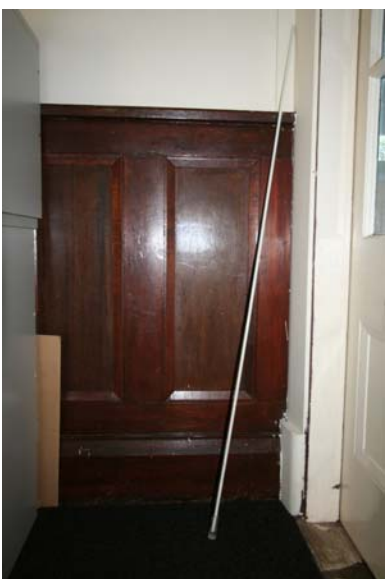
Photograph 84 Retained dado wall panel with original finish
