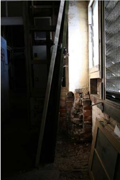
Photograph 16 Former laundry – modified and High significance
