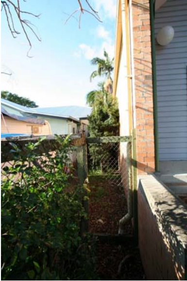
Photograph 43 The extension: Fabric and details – Moderate significance
