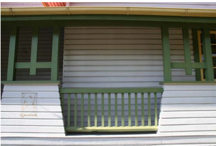
Photograph 39 Original fabric and details – Exceptional significance
