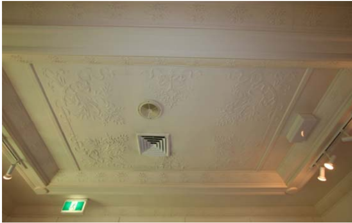
Photograph 1 The original ceiling – exceptional significance
