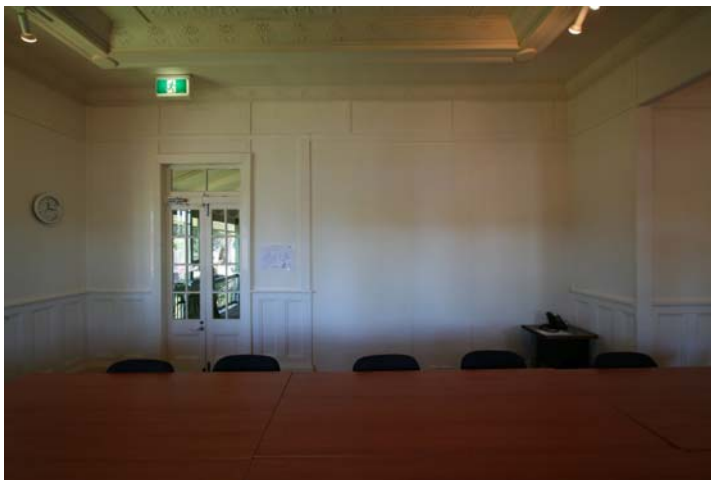
Photograph 3 original waist high panels and modified elements – High level of significance
