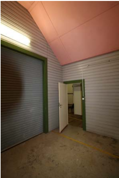
Photograph 139 Enclosed loading dock
