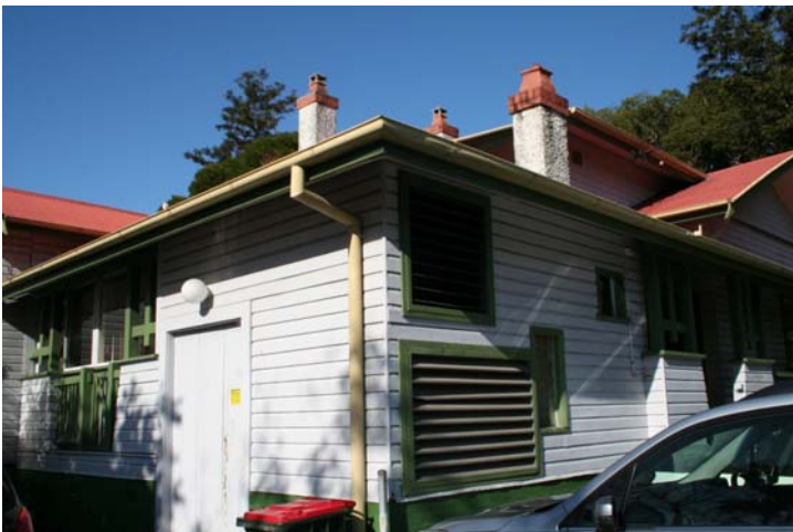
Photograph 23 Former laundry – Modified and Moderate significance
