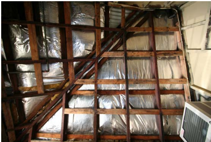
Photograph 11 Modified store-room roof – Moderate significance
