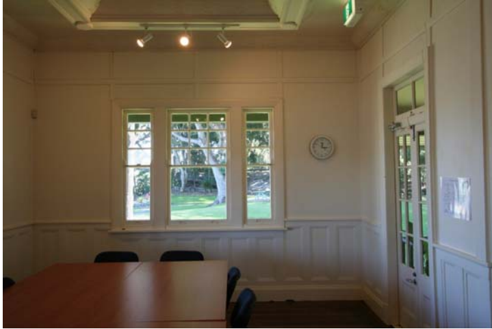
Photograph 4 Original windows and panelling – Exceptional significance
