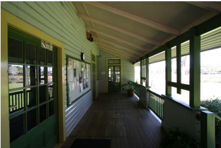
Photograph 20 Front verandah– modified but original fabric and Exceptional significance
