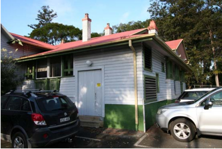
Photograph 64 The Laundry enclosure
