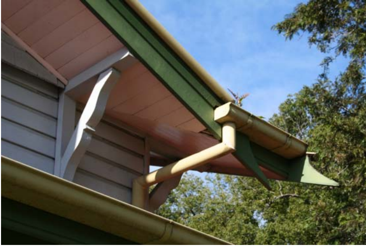
Photograph 37 Original fabric and details – Exceptional significance
