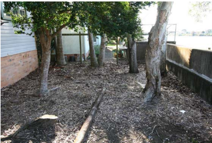
Photograph 62 The north eastern corner behind the flood wall
