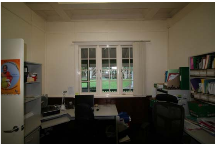
Photograph 78 The original dado level wall panels
