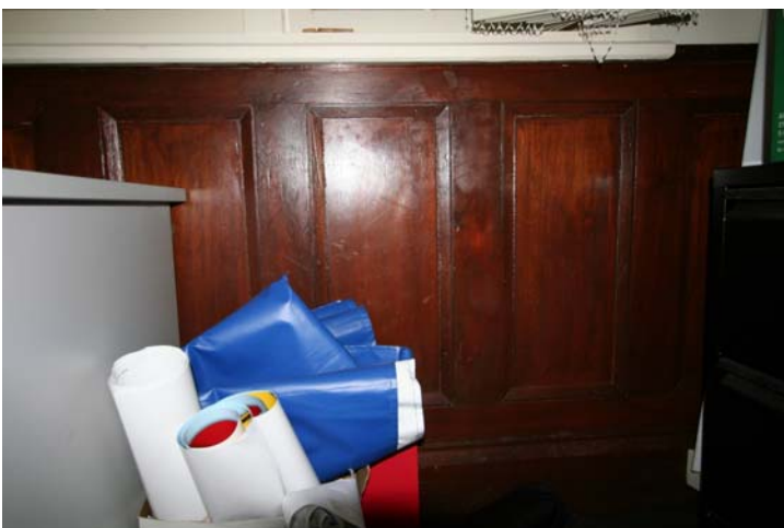
Photograph 75 The original finish on the wall dadao panels
