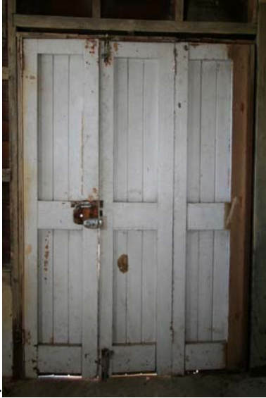
Photograph 10 Original doors – High level of significance
