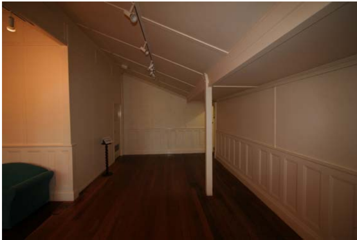
Photograph 147 The former rear verandah with bulkheads and post retained and relocated dado panels
