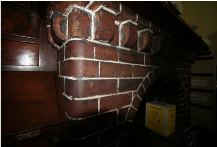
Photograph 80 Brick fireplace details
