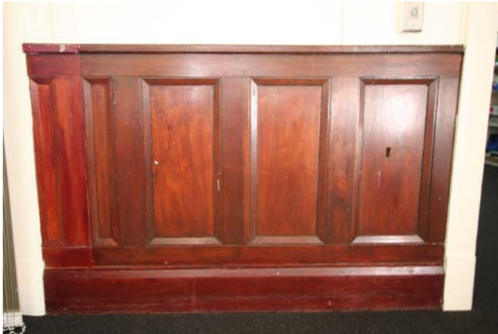
Photograph 85 Retained dado wall panel with original finish
