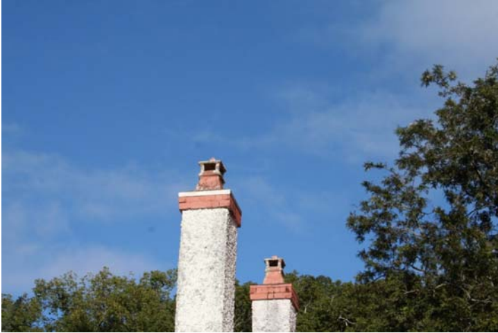
Photograph 40 Original fabric and details – Exceptional significance
