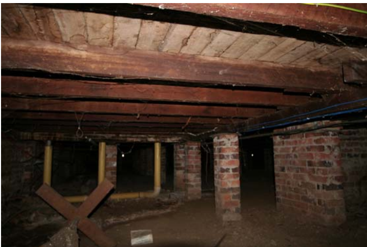
Photograph 9 Sub-floor view indicating generally sound conditions
