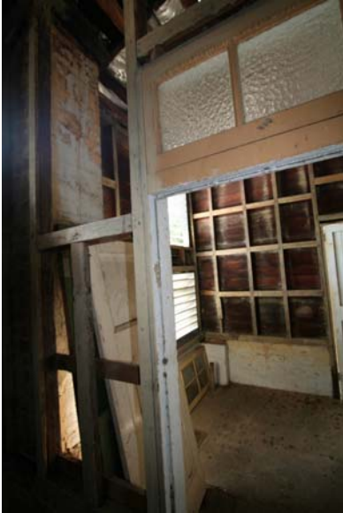
Photograph 13 Former laundry – modified and High significance
