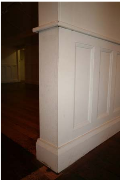
Photograph 145 Post enclosed in modified wall treatment
