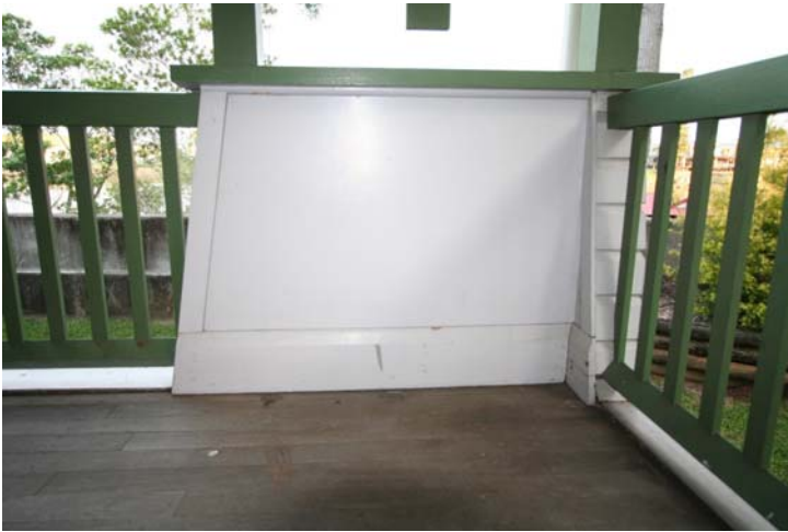
Photograph 68 Verandah detail showing the sheet clad piers
