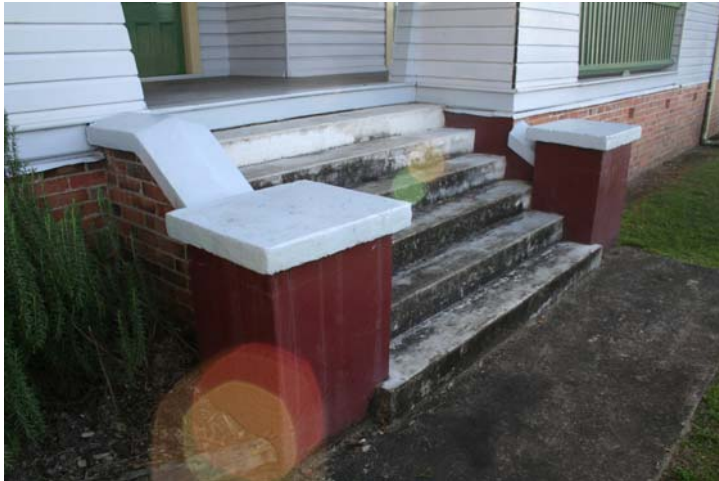
Photograph 31 Original fabric and details – exceptional significance
