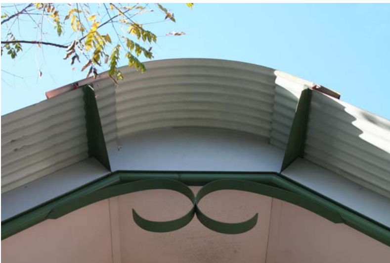
Photograph 42 The extension: Fabric and details – Moderate significance
