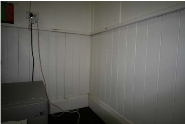
Photograph 92 Unusual half timbered dado area within the secondary and service areas of the former residence
