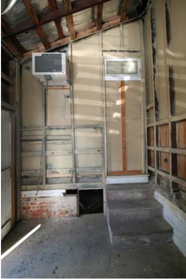
Photograph 19 Former laundry – modified and High significance
