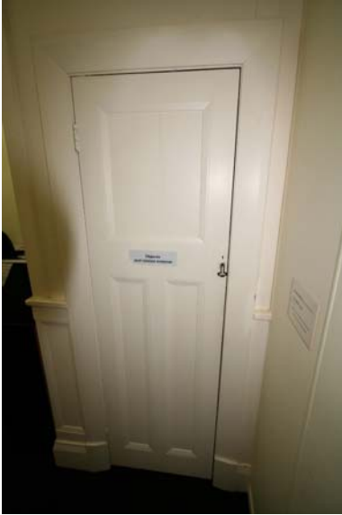
Photograph 112 Exceptional built in cupboard
