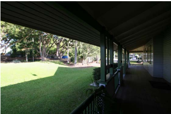
Photograph 57 Exceptionally significant front western verandah – lost front steps
