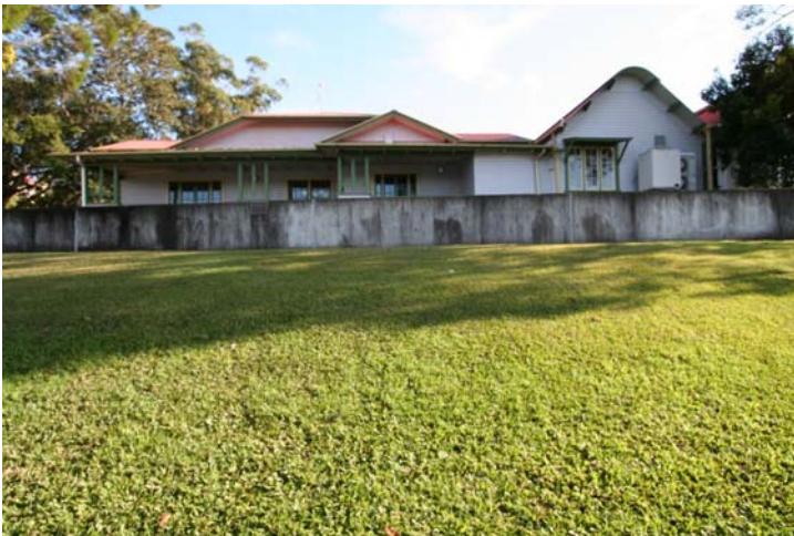
Photograph 50 The extension: Original fabric and Extension fabric and details – Moderate & Intrusive significance
