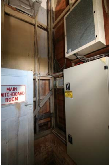
Photograph 15 Former laundry – modified and High significance
