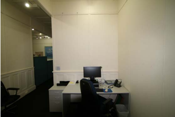
Photograph 117 Retained bulkheads define the former central passage of the residence. Note partition in plasterboard without dado panels
