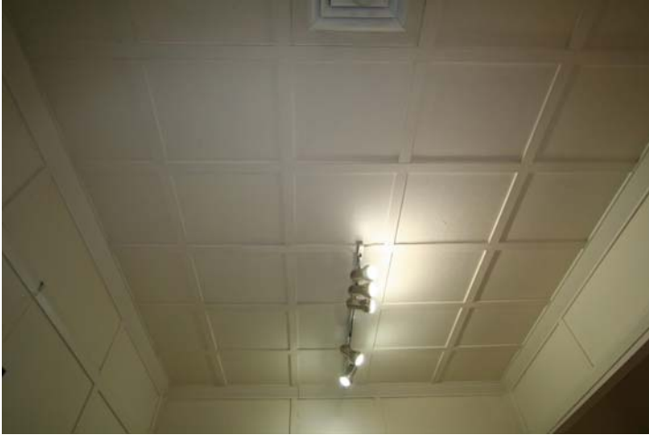
Photograph 109 The distinctive ceiling, cornice and bulkhead and the ineffective former gallery lighting
