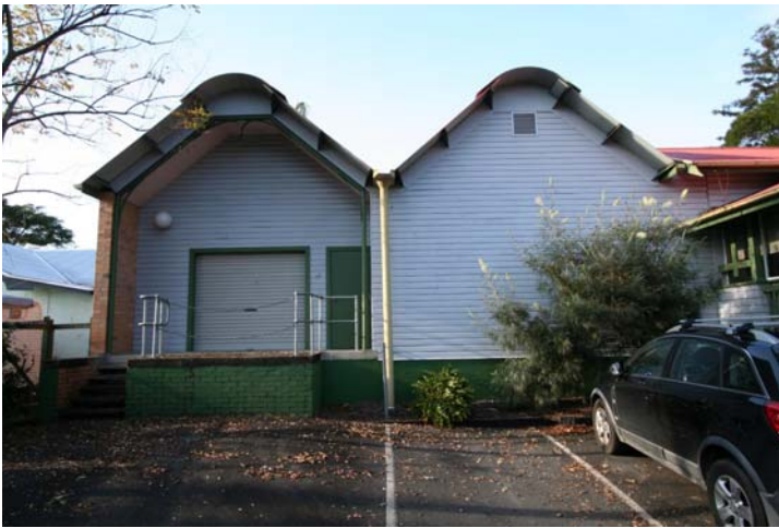
Photograph 65 The sensitive 1988 extension – North eastern corner
