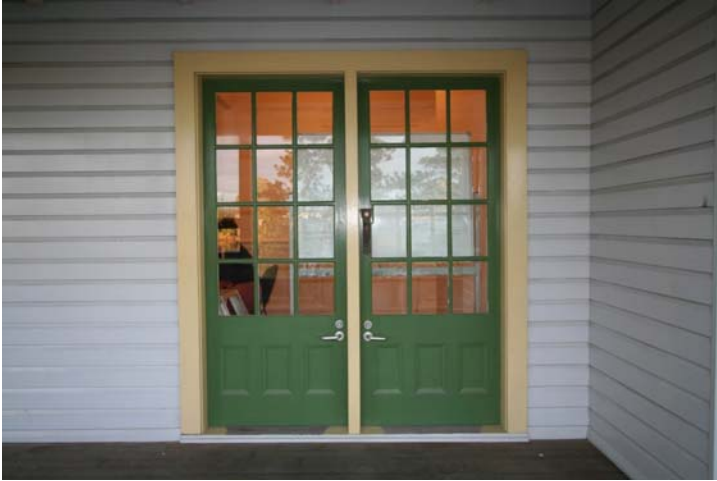
Photograph 70 Contemporary but sympathetic door set to verandah
