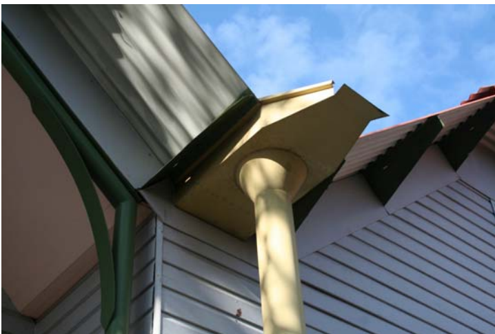
Photograph 41 The extension: Fabric and details – Moderate significance
