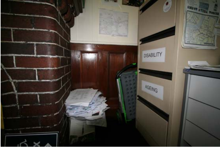
Photograph 76 Original face brick fireplace and dado wall panels
