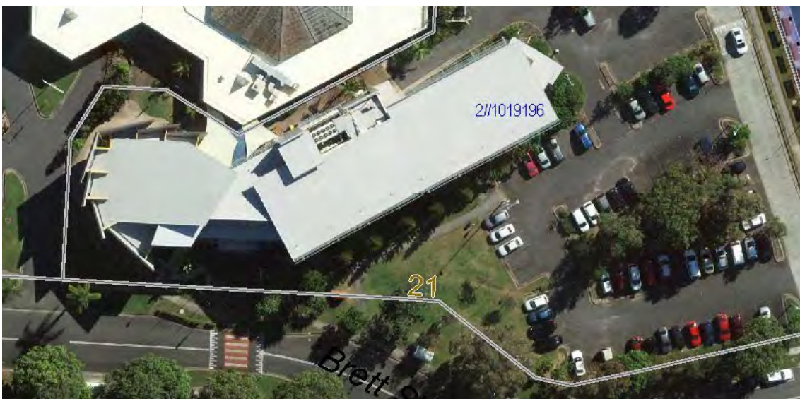
Photo 2 - Aerial View of Existing Building
