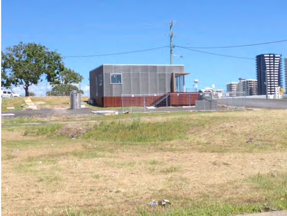
Photo 2 - Construction stage (15 January 2015)
