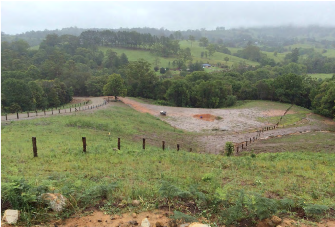
Photograph 13 - Provided by site owner to NSW Crown Lands 5 January 2015. No commentary provided with this photos. The photo demonstrates good grass coverage on previously exposed batters.
