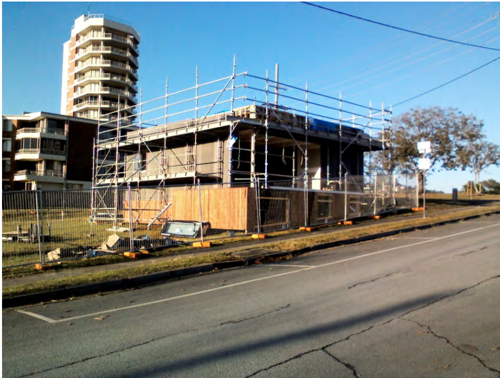
Photo 1 - Construction being undertaken (20 November 2014)
