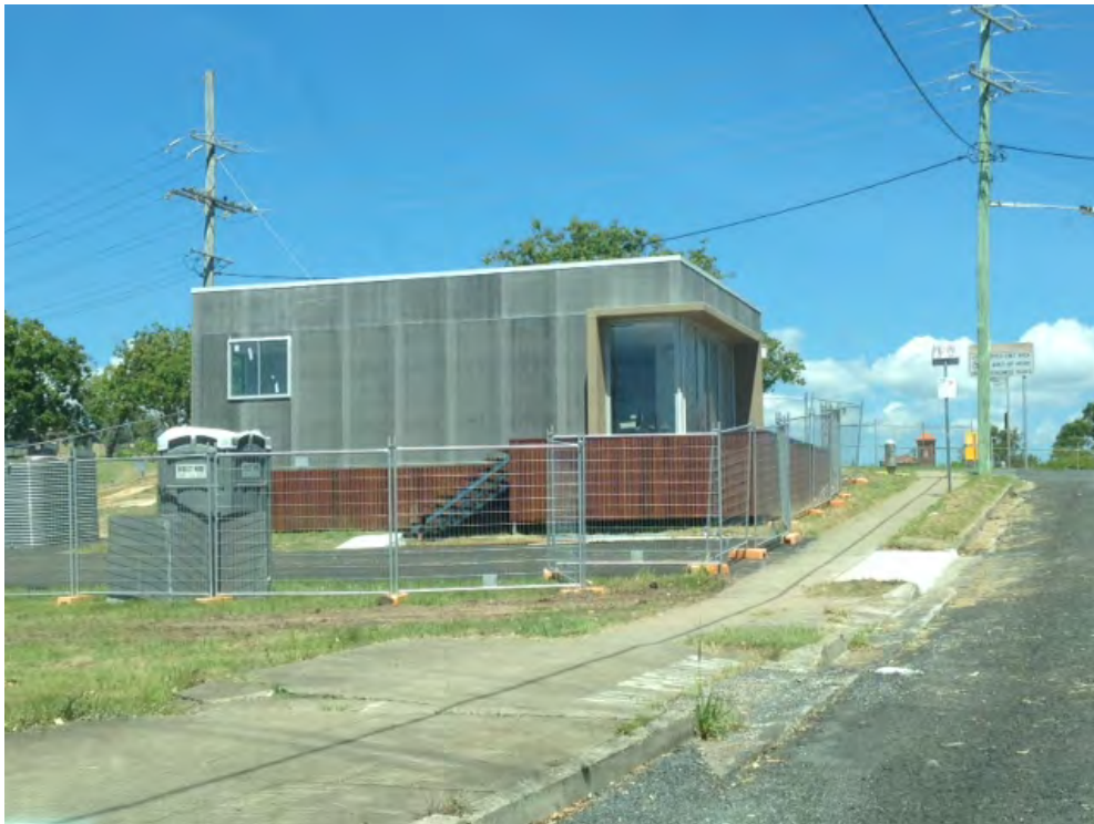
Photo 3 - Construction stage (15 January 2015)
