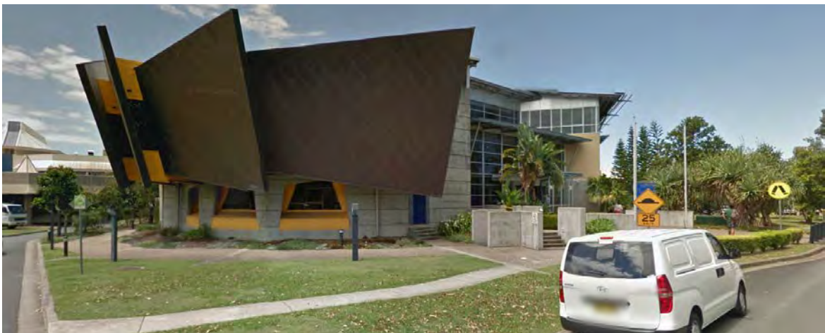
Photo 1 - View looking east along Brett Street of existing Building
