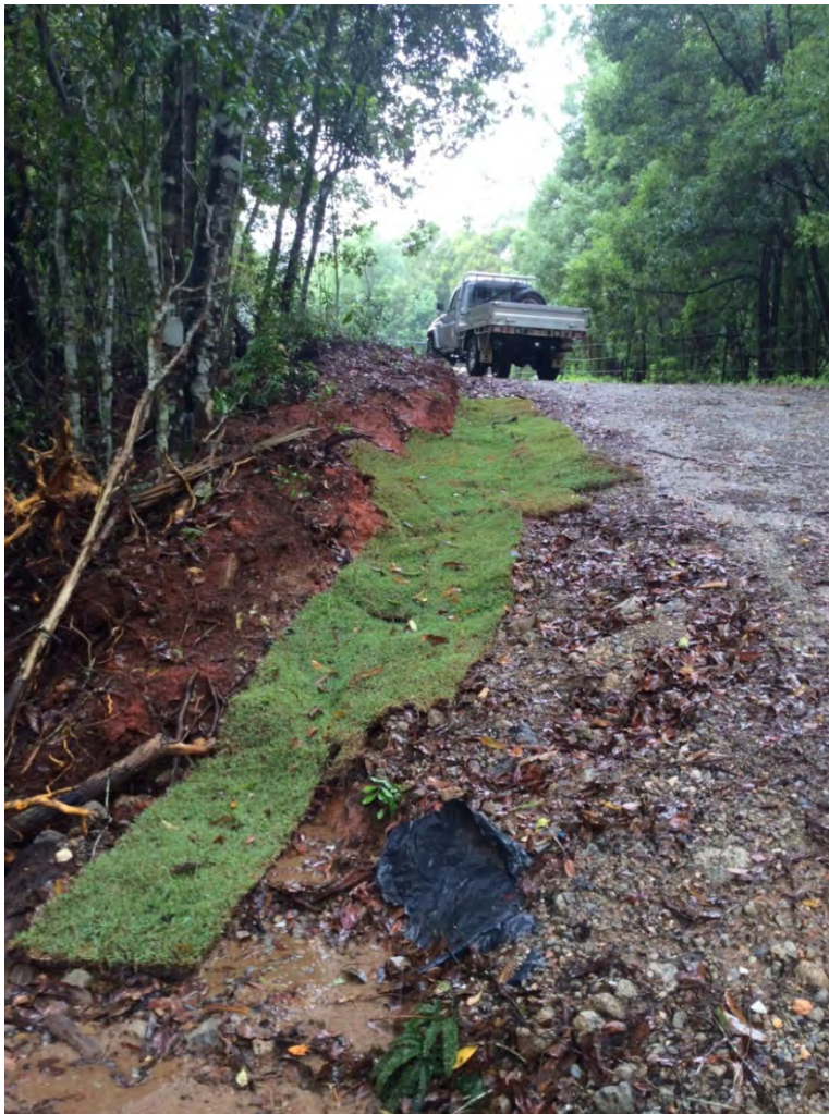
Photograph 6 - Provided by site owner to NSW Crown Lands 5 January 2015. Indicates turf has been laid near the entry gate.
