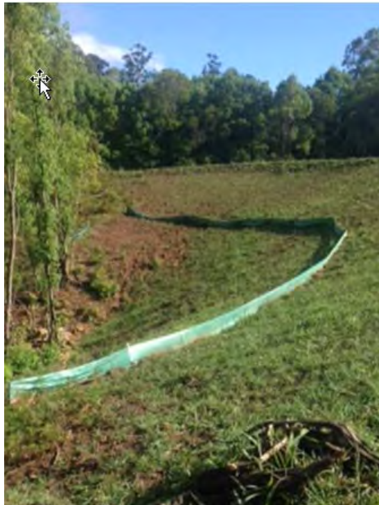
Photograph 1 - Existing sediment and erosion controls maintained. Build up of sediments from previous rain event have been removed. Significant grass cover has established on previously exposed batters.
