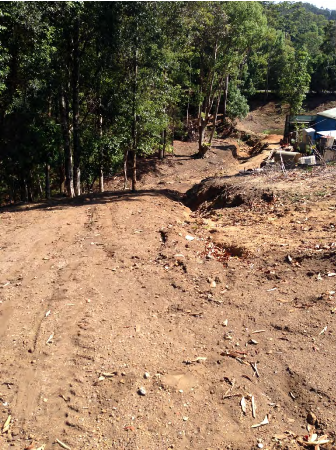
Photo 2 - Drainage line adjacent to water course that improved sediment and erosion control practices were identified to be established.
