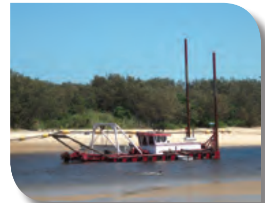
Sand dredging at Kingscliff.
