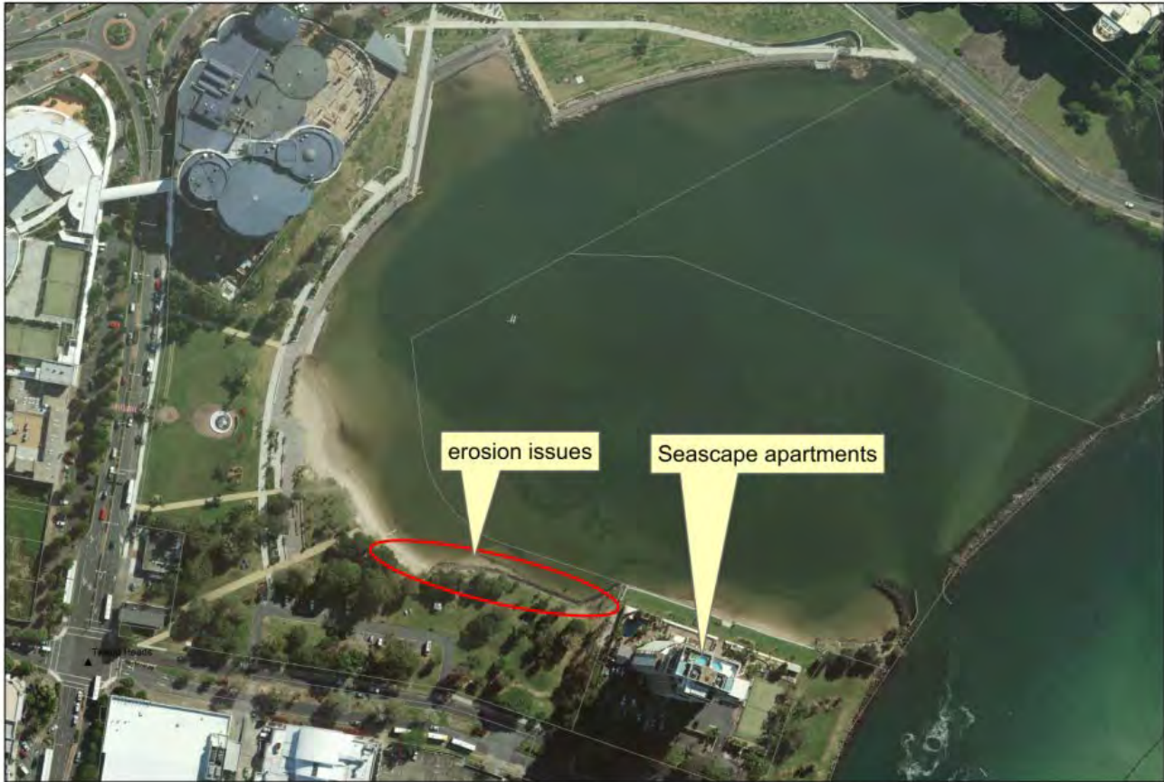
Jack Evans Boat Harbour - southern beach erosion area
