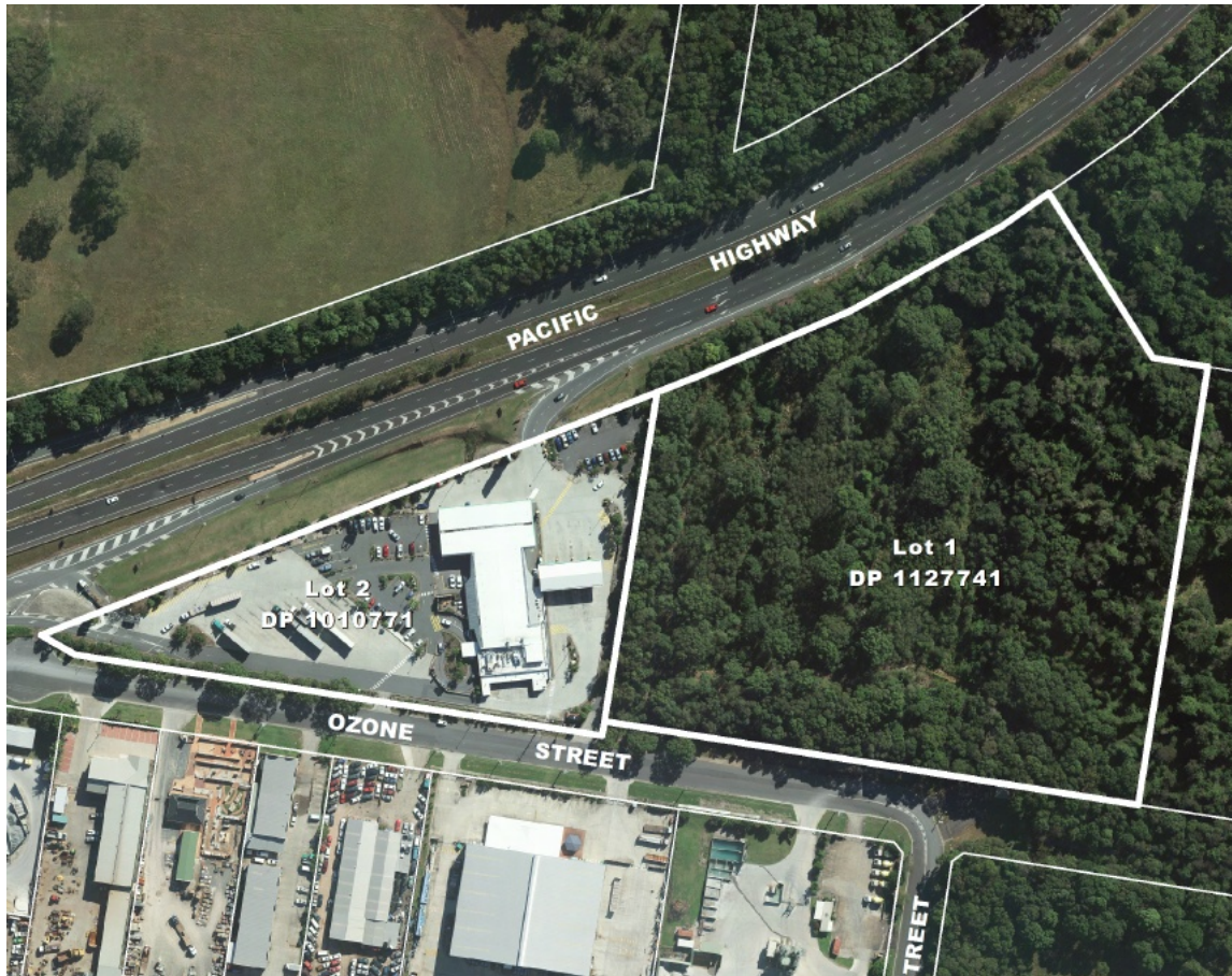
Fig 1. Location of the BP highway service centre.
