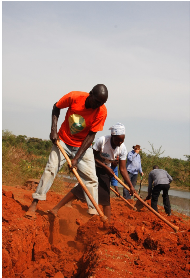
Installing the pipeline to Manyasi Dam kiosk
