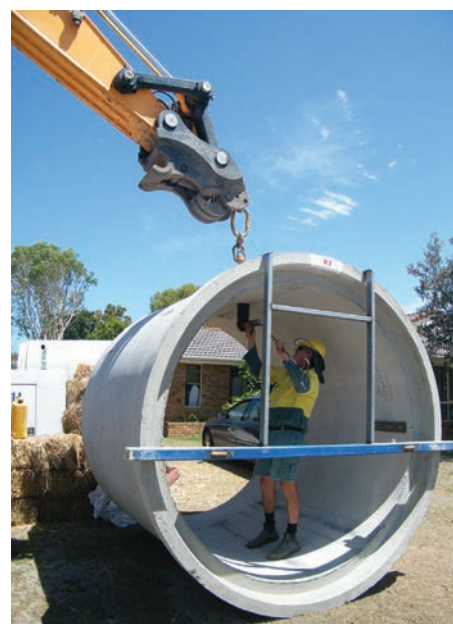
Hooking up stormwater pipes being laid at Blue Jay Circuit Kingscliff
