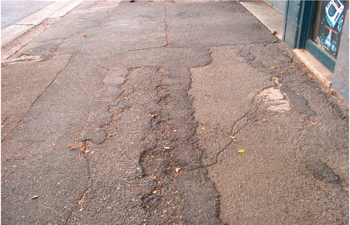
Figure 6 – Example Concrete Footpath Condition Score 3
