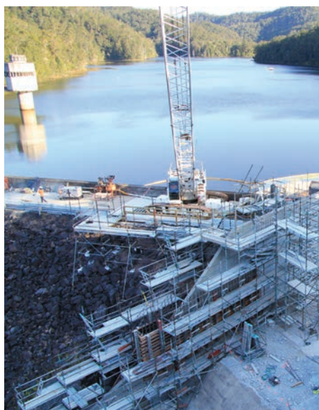
Clarrie Hall Dam Spillway Upgrade
