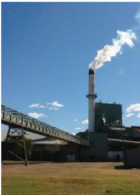
Condong Sugar Mill and cogeneration plant
