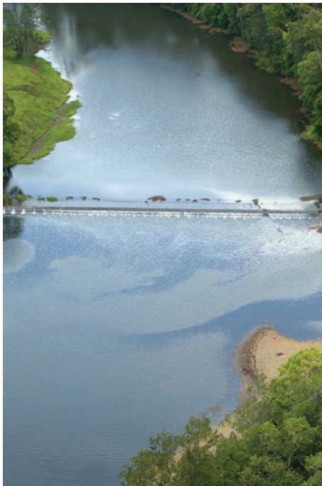
Bray Park weir
