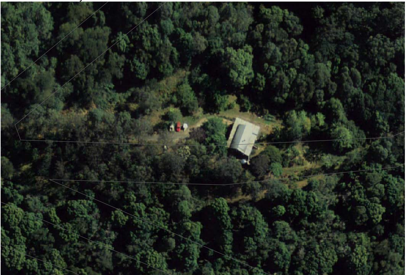
Structure in vicinity of road reserve:-
