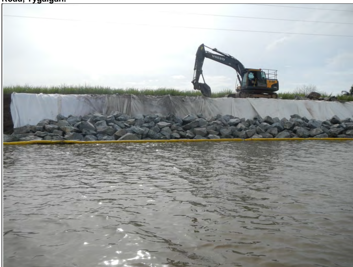
Figure 2. Reactive river bank erosion stabilisation works being constructed adjacent to Tumbulgum Road, Tyngalga.
