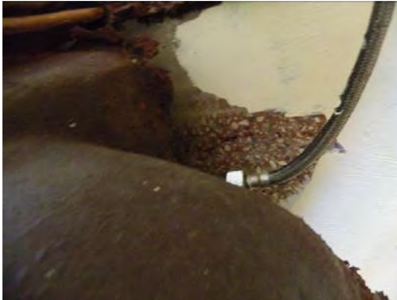
Figure 11: Terrazzo flooring showing successive new layers laid over original.
