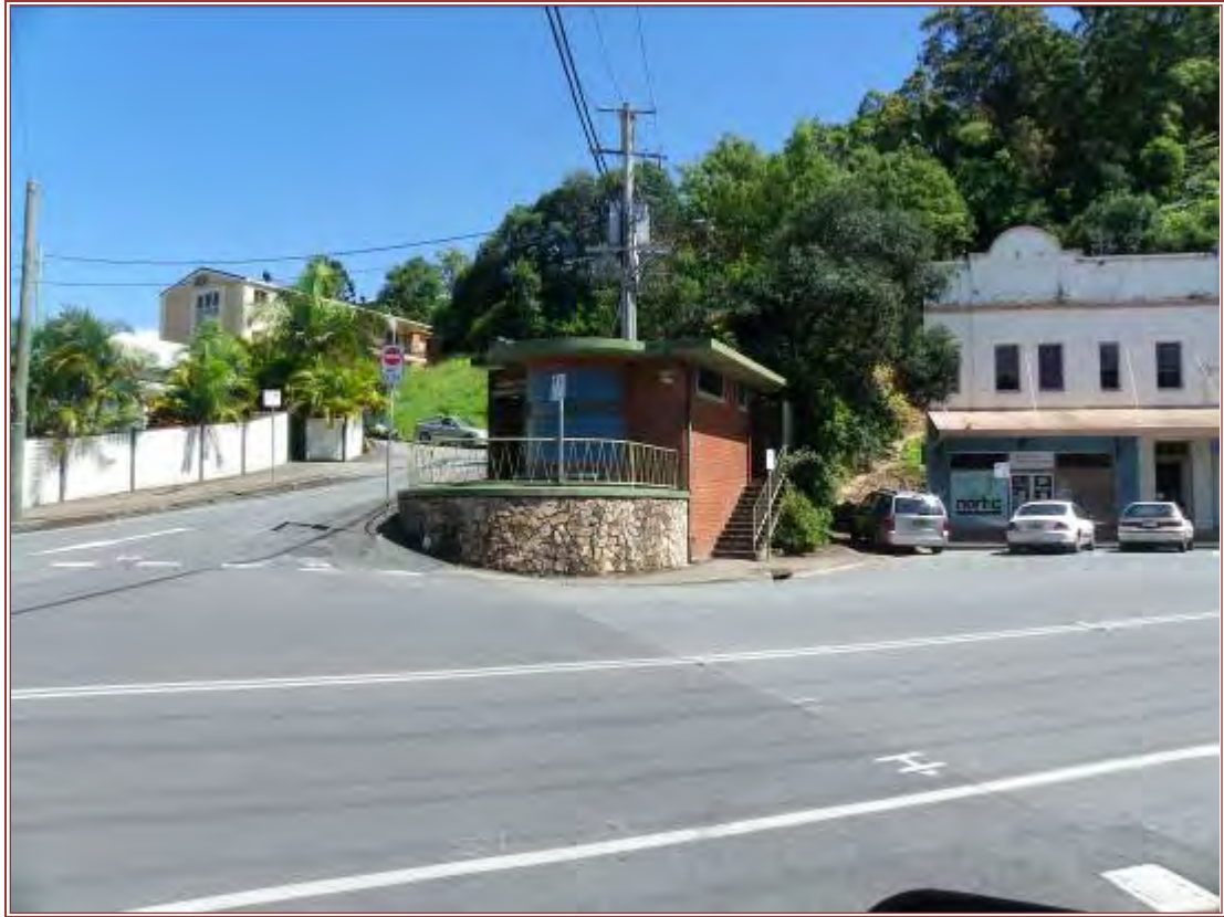
Figure 2: Main elevation of the site.
