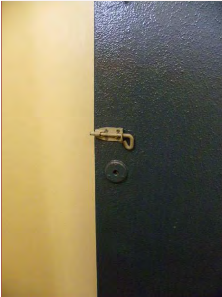
Figure 9: Original doors with marks of original fittings.
