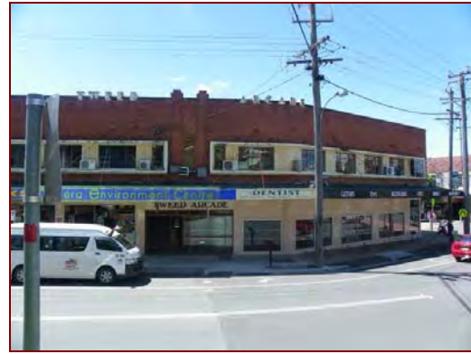
Figure 2.47: Tweed Arcade viewed from the Toilet Block.
