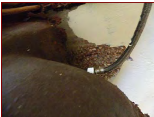
Figure 2.44: some of the original terrazzo visible behind the basin in the men's toilets.
