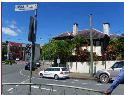
Figure 3.6: View to the south-west.
