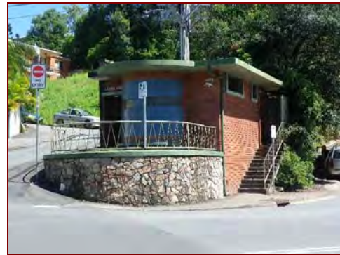
Figure 3.15: Southern elevation showing the retaining wall
