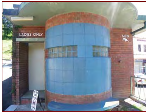
Figure 3.14: Southern elevation, dominated by the semi-circular bay.
