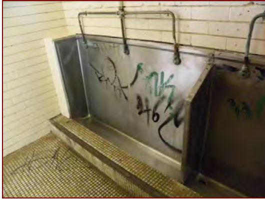
Figure 2.42: Men's urinal, note the original water spouts
