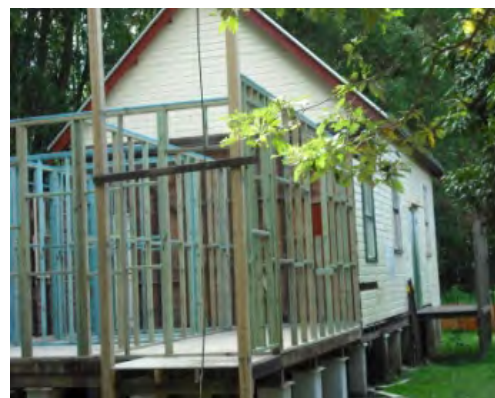
New extension, toilets and kitchen
