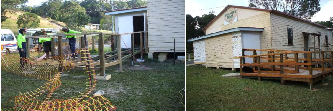
Piggabeen Hall ramp construction
