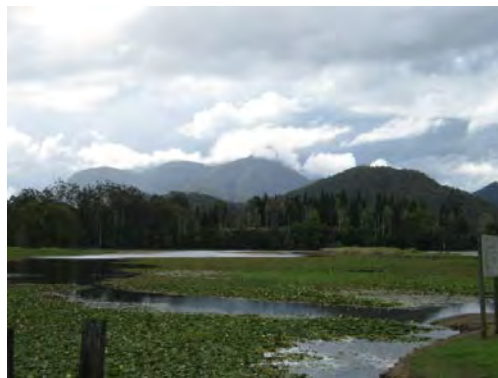
Clarrie Hall Dam
