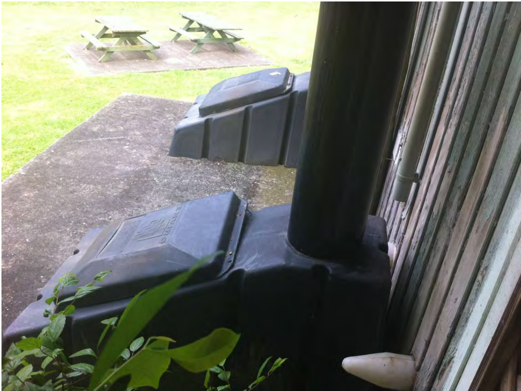
Photo 9 Compost chamber manholes.
