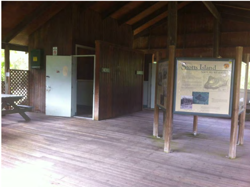
Photo 10 View of toilet facilities and undercover area.
