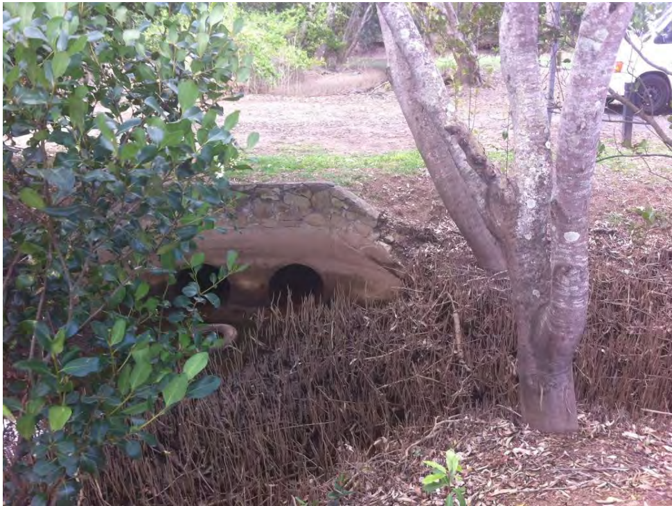
Photo 3 Existing stormwater culvert approximately 10m north of available LAA. Discharges directly to Tweed River and is impacted by tidal movement.
