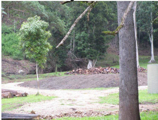
Photo 6 - towards cut building pad
