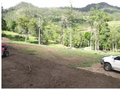
Photo 2 - excavated pad (looking south west)
