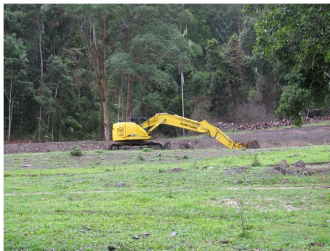
Photo 4 - looking east towards subject site
