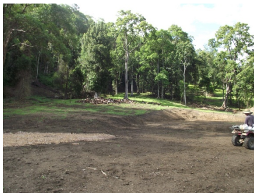
Photo 1 - excavated pad towards existing vegetation (looking east)
