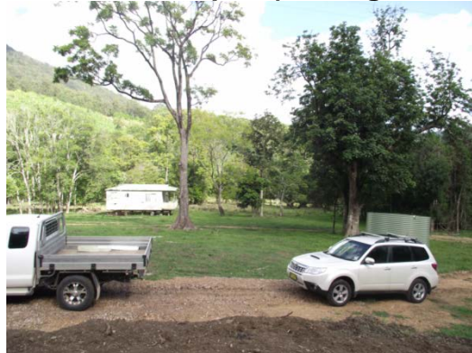
Photo 3 - looking from building pad to west
