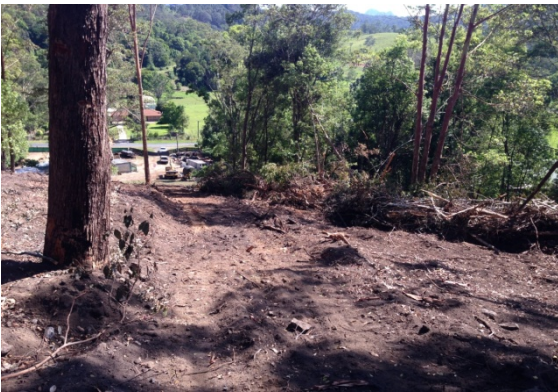
Photo 1 - Approximately 100m of regrowth vegetation has been cleared.
