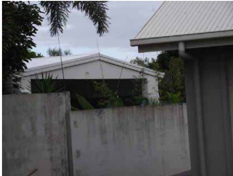
Close up of corner of garage at 9A Ulladulla Court, showing proximity to 12 Cactus Court deck and entertaining area. The pool is to the left of the structure.
