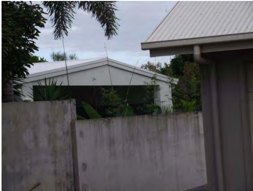
Close up of corner of garage at 9A Ulladulla Court, showing proximity to 12 Cactus Court deck and entertaining area. The pool is to the left of the structure.
