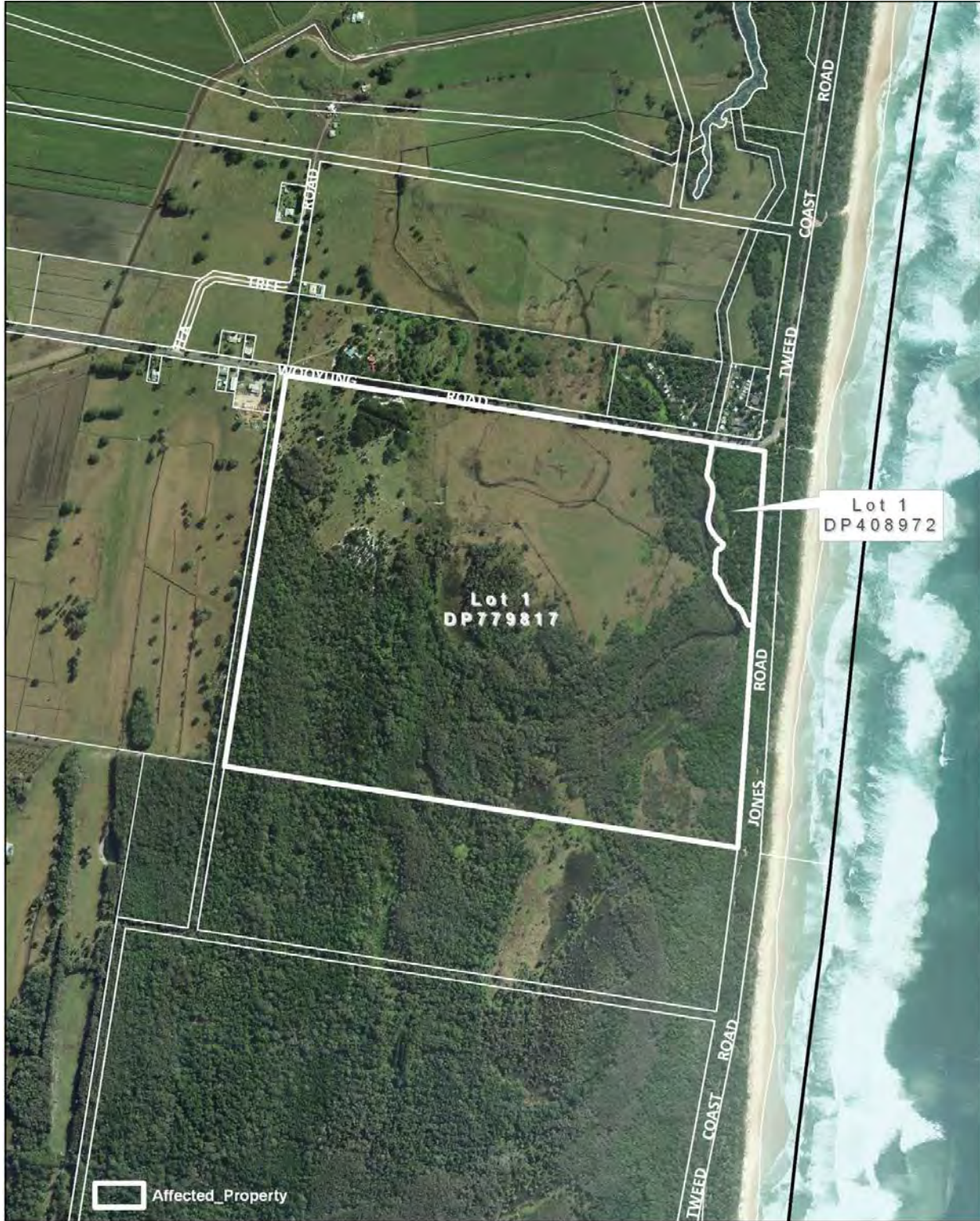
FIGURE 2: AERIAL IMAGE OF SITE - 2012
