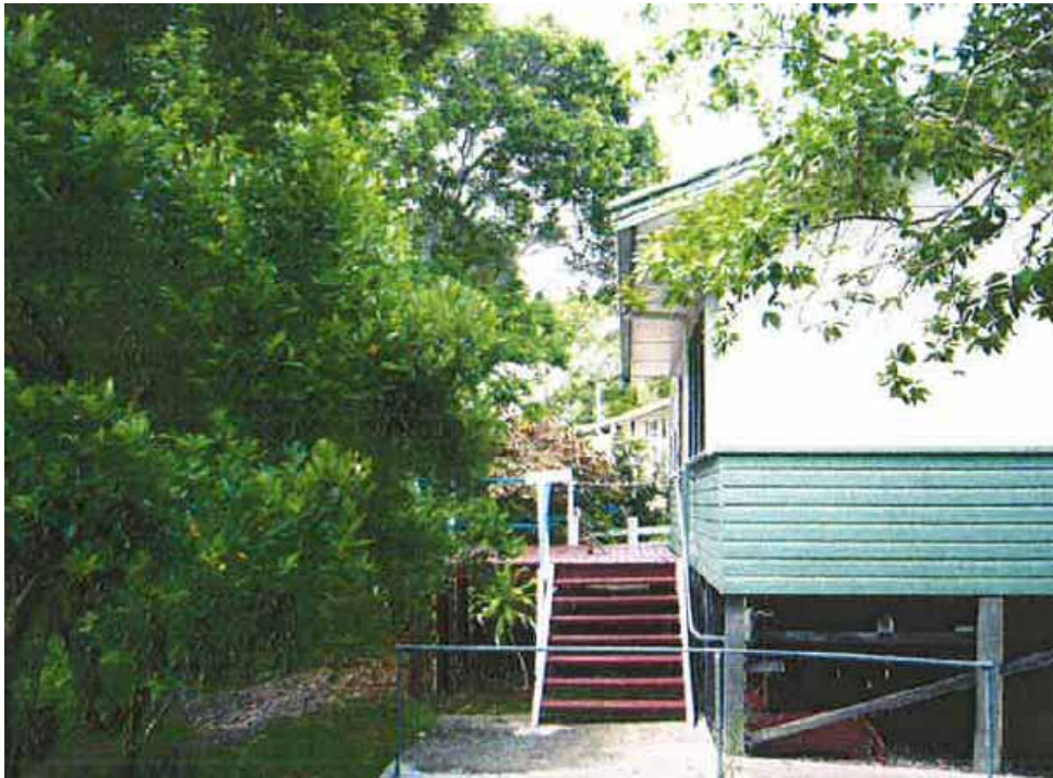
Figure 11: deck addition at rear encroaching into public reserve
