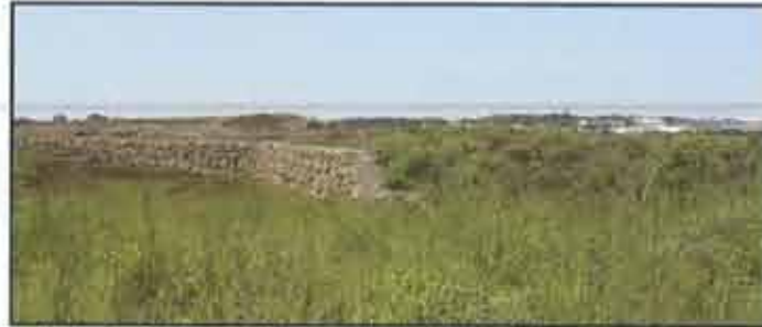
Photo 3: Existing retaining wall in the North of the subject site
