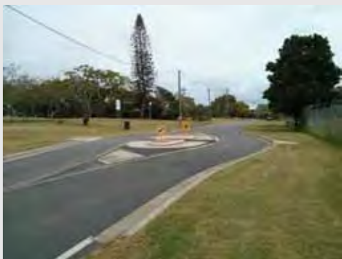
Pedestrian refuge crossing on River Street
