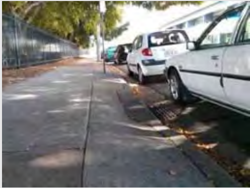
Kerb angle and side entry pit on Stuart Street
