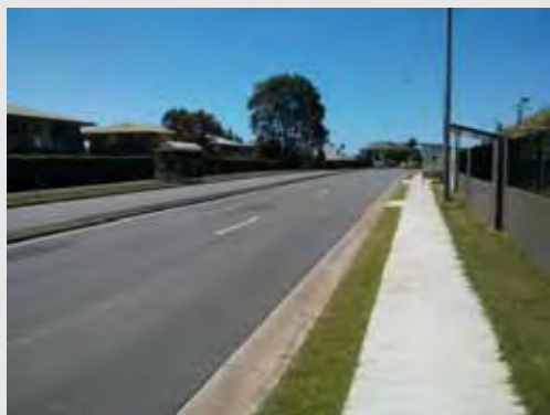
Bus stops and median on Darlington Drive
