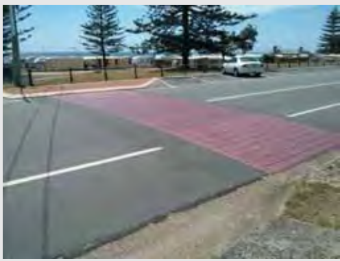
Pavement treatment on Marine Parade
