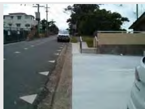
Stairs on Bent Street
