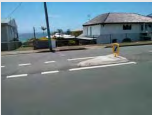
No footpath on northern side of Sutherland Street
