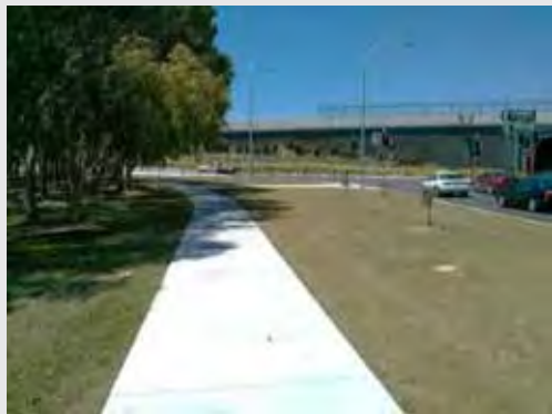
Darlington Drive shared path on approach to Sexton Hill Drive
