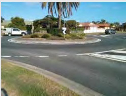
Darlington Drive/Woodbridge Drive roundabout
