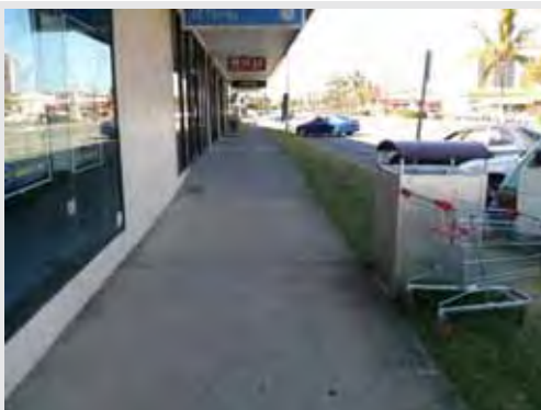
Steep grade transition on Wharf Street
