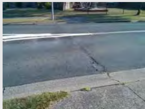
Narrow roundabout splitter island, lack of kerb ramps at Darlington Drive/Woodbridge Drive roundabout
