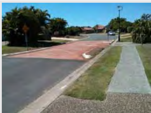
Pavement treatment (slow point) on Avondale Drive
