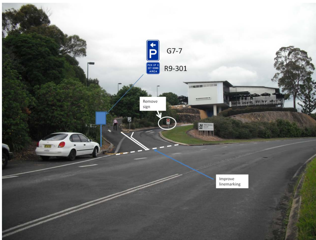
Figure 4 - suggested signage and linemarking changes
