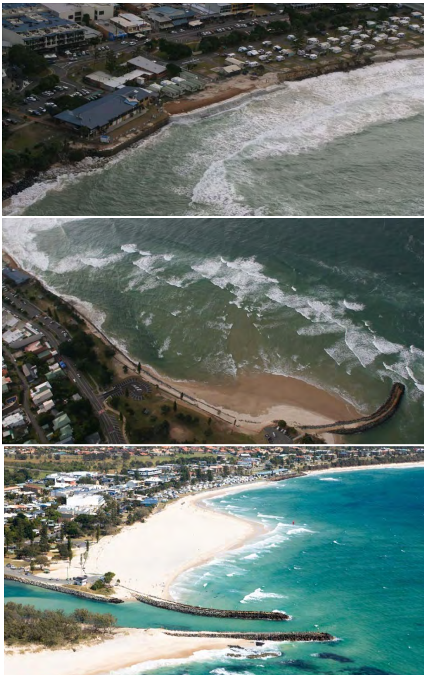
Figure 4-5 Kingscliff erosion in August 2011 (top; mid) and recovery to 2012 (bottom)
