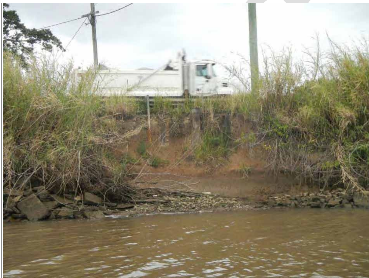
Figure 3. Bank slip adjacent to the Tweed Valley Way near Stotts Island. Road safety barrier anchor posts can be seen exposed in the top of the bank.
