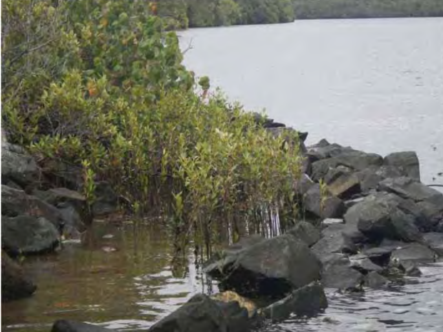
Figure 4. Rock fillets constructed at Chinderah, with regenerating mangroves.
