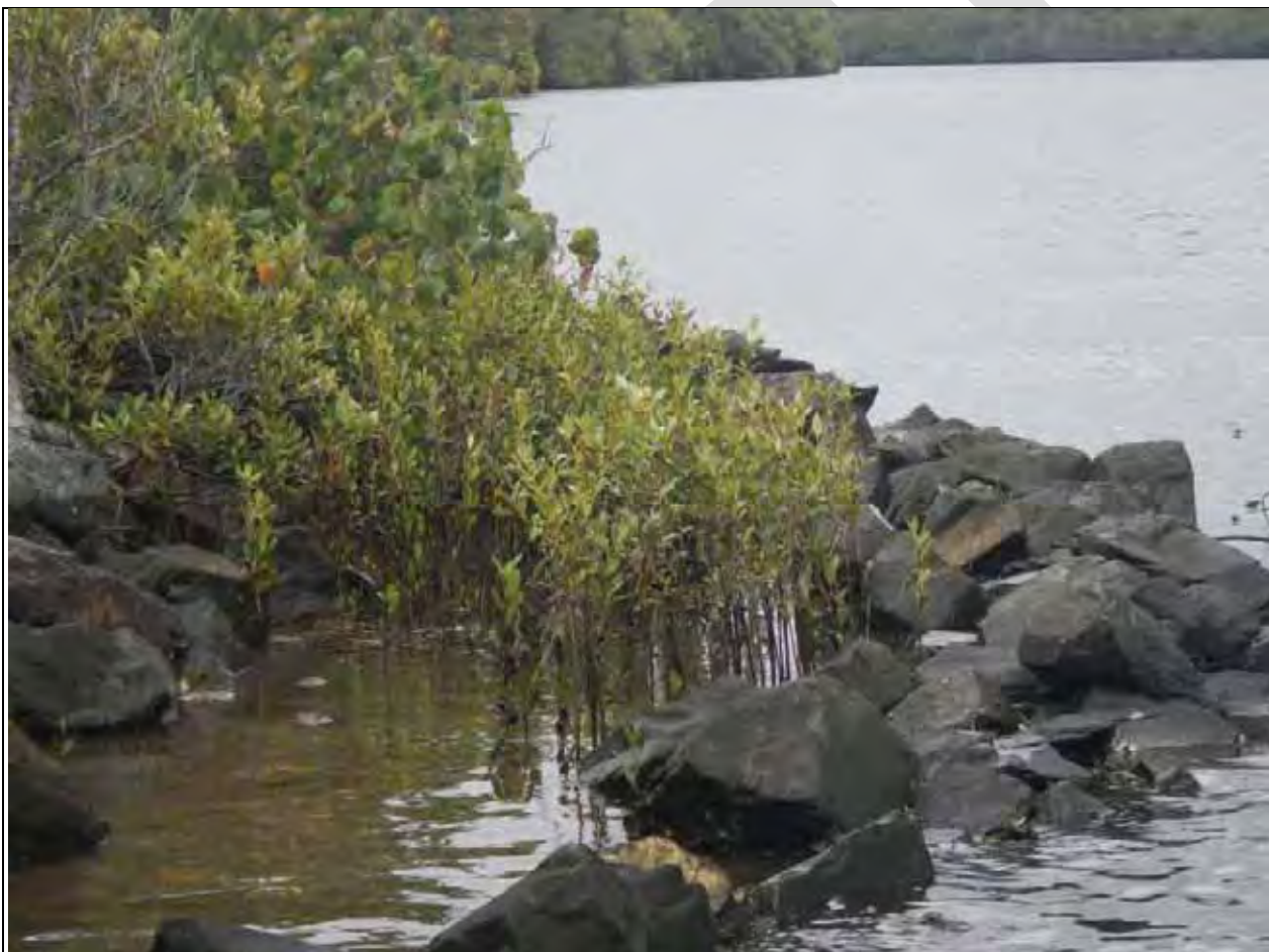
Figure 2. Rock fillets constructed on Chinderah bay drive showing natural mangrove recruitment. This area provides excellent fish habitat, a high level of erosion protection and will eventually have a very low visual impact.
