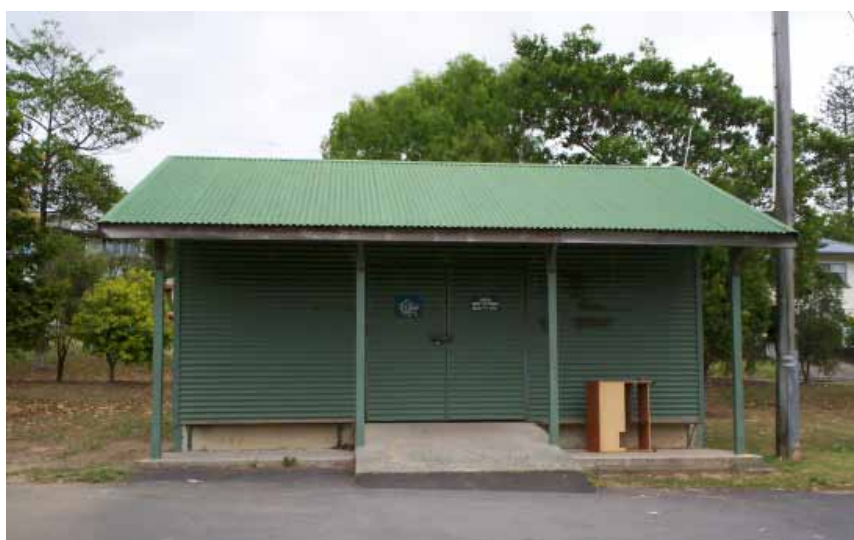
Figure 2: Existing Council shed utilised for Men's Shed activities
