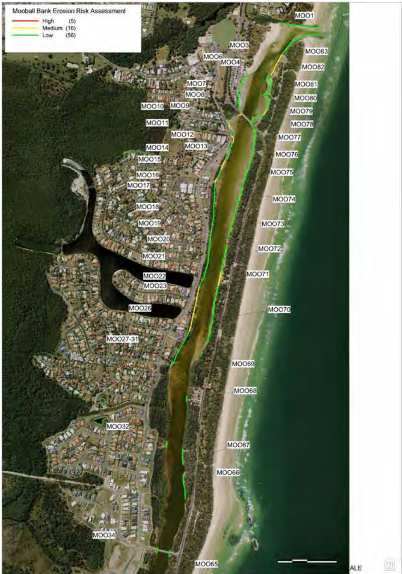
Figure 15: Mooball Creek Bank Erosion Risk (refer Appendix 3 for further details)
