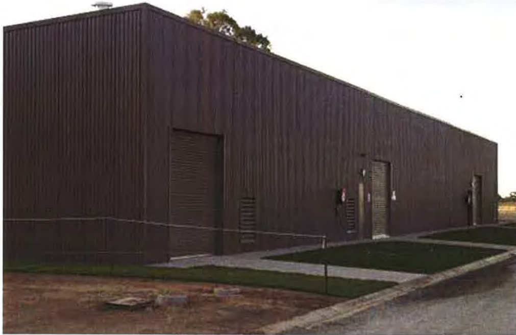
Figure 5-5: Existing treatment plant building at Deep Creek Marina NSW.
