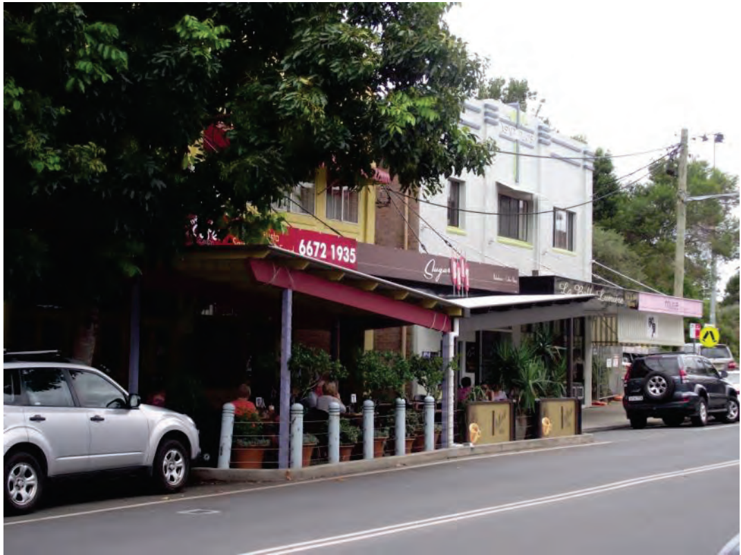
Outdoor dining area and awning structure within road reserve at the Sugarbeat Cafe, Commercial Road
