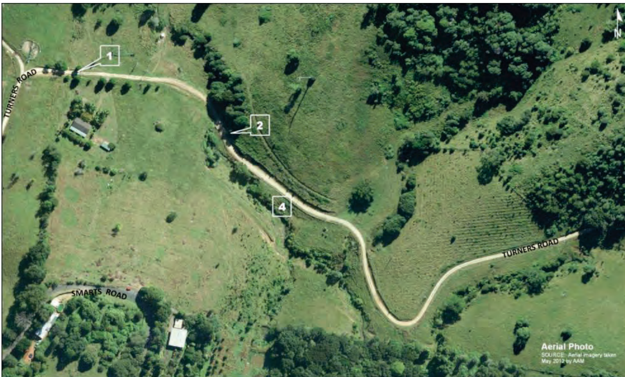
Figure 3 - Aerial photo below showing the locations of the alleged unauthorised uses and works on the adjoining Crown road reserve and Right of Way, and within the premises, No. 140 Turners Road.
