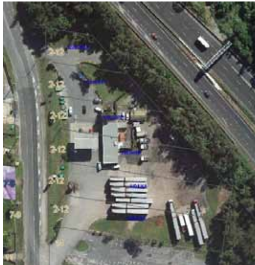
Figure 2: Aerial view of BP Chinderah Car parking area
