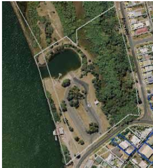
Figure 1: Aerial view of Fingal Head Boat Ramp site
