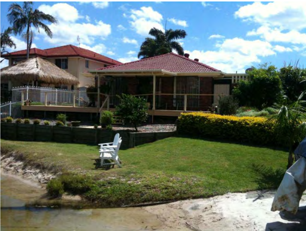
The above photograph indicates two neighbouring properties to the north west of the subject property.
