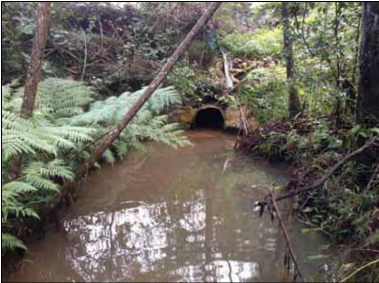
Plate 1: Outlet of piped section of the subject creek.
