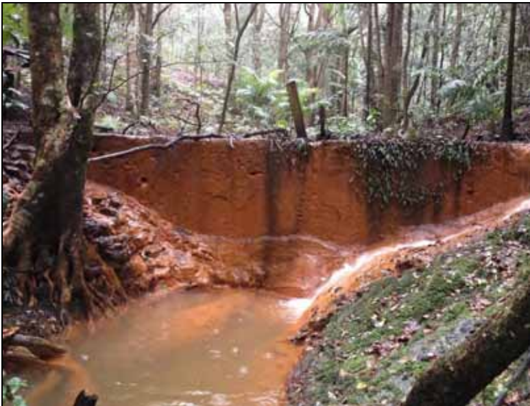
Plate 2: Constructed weir located midway between the culverts at Harrys Road and Kinnears Quarry (note iron staining on concrete surfaces; Fish and crustaceans were observed in the pools directly below the weir)
