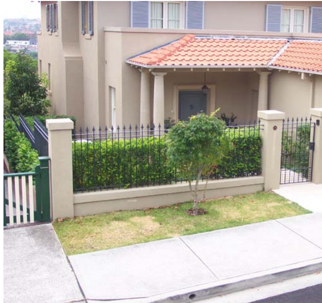
This fence returns down the side boundary, combines landscaping, open fencing and low walls to create a fence that enhances the pedestrian scale and residential qualities of the street.
