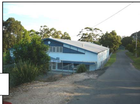
Plate 4. View south down Adelaide Street to existing P&CY Club building.
