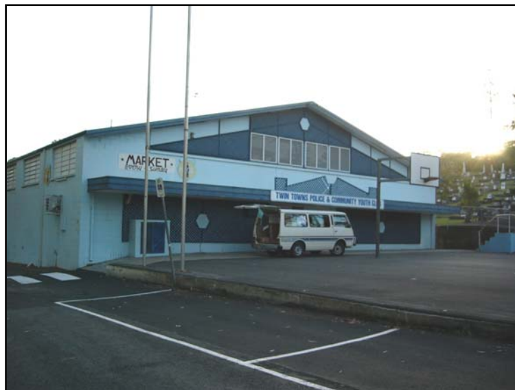
Plate 6. View from internal road entry on Florence Street to existing P&CY building.
