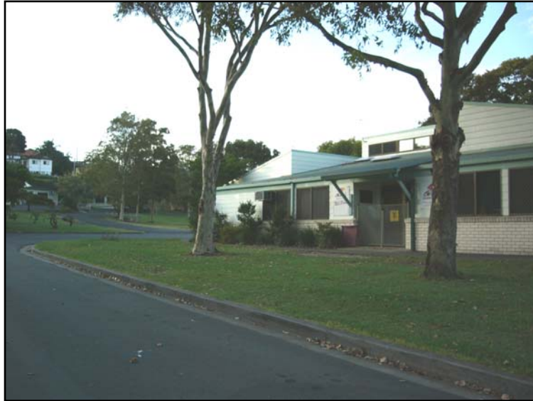
Plate 9. View northwest from entrance of internal road off Recreation Street to existing child care centre.
