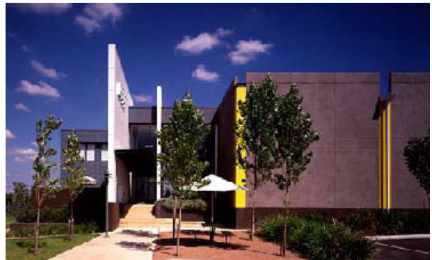
ii. Building legibility defined by architectural elements, colour and light.
