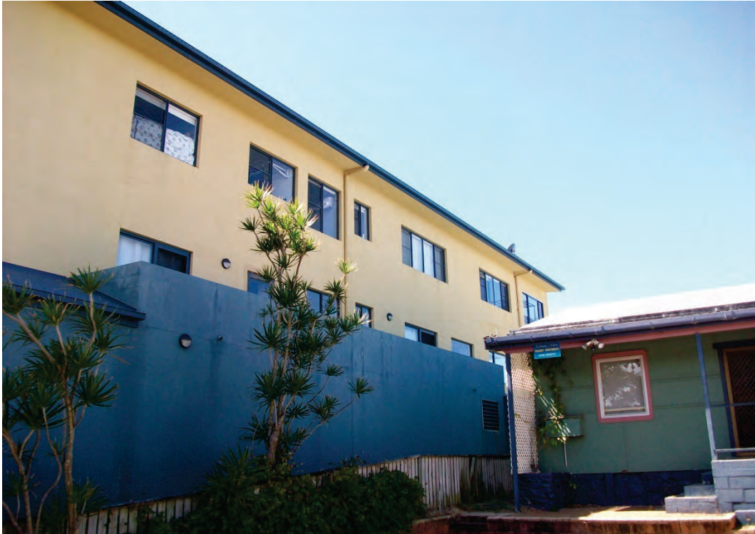
Figure 9 View of adjacent three storey units.
