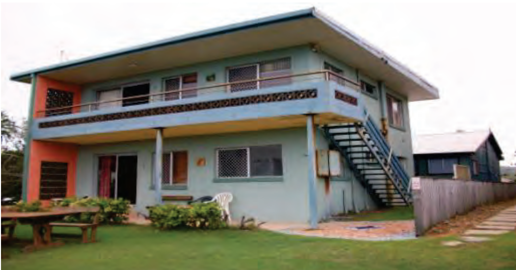
Figure 4-West view of existing units foreground building to be partly retained
