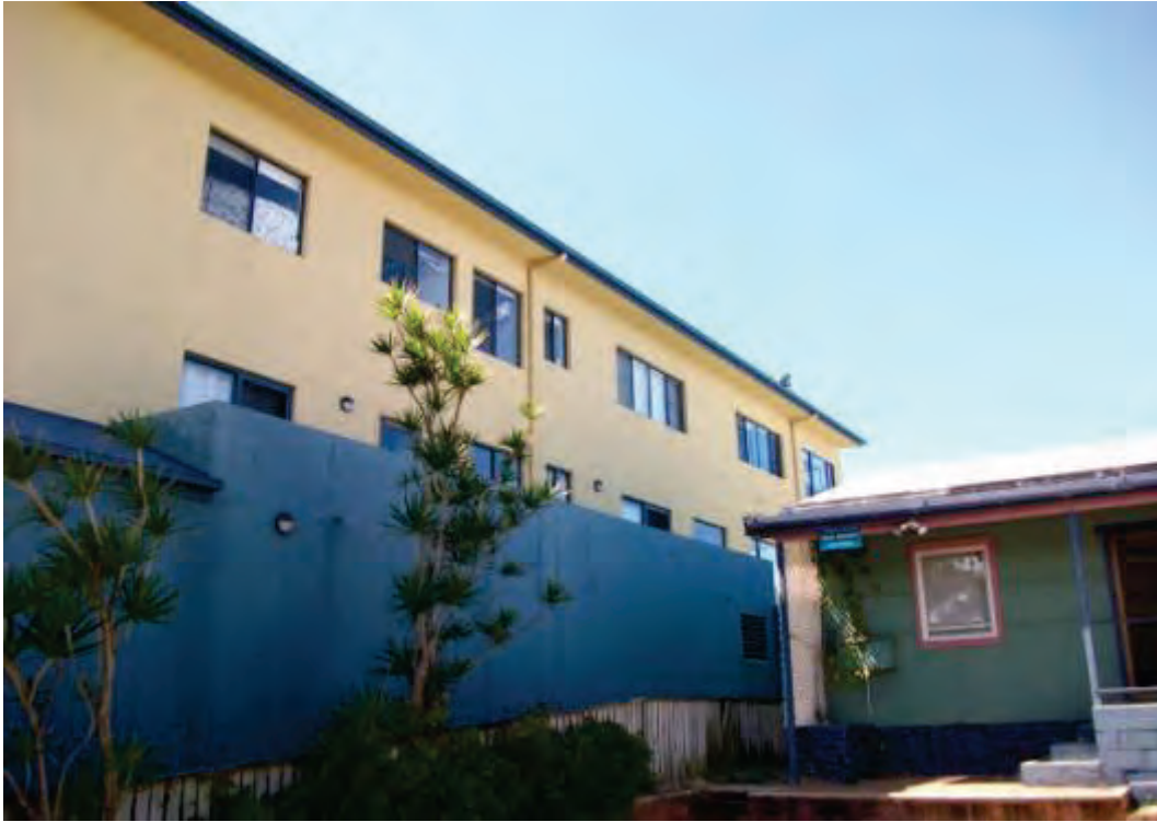
Figure 9 View of adjacent three storey units.
