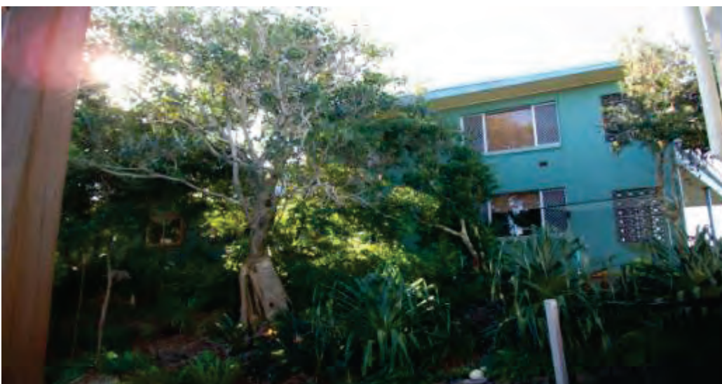
Figure 5- view north from dwelling entry of adjoining property to south
