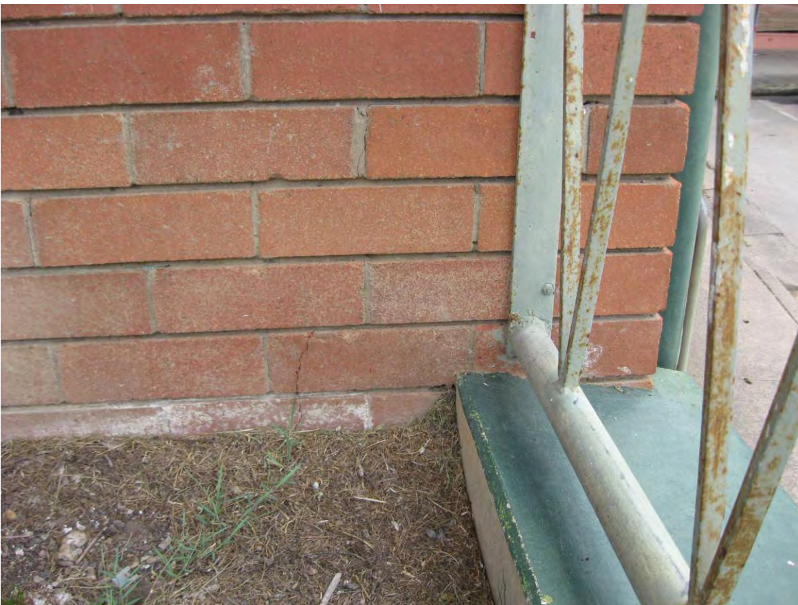
Figure 6 – South east corner
