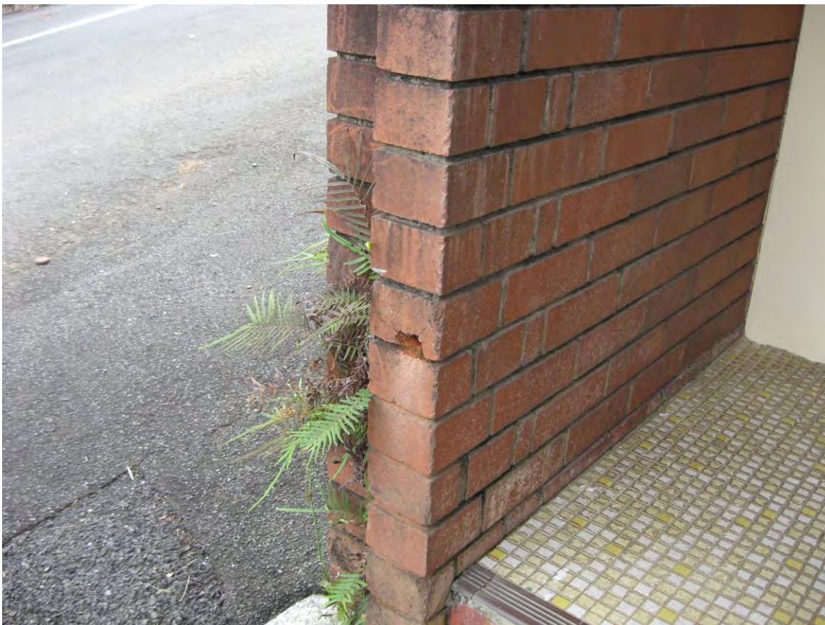
Figure 10 – Bolt damage to doorway
