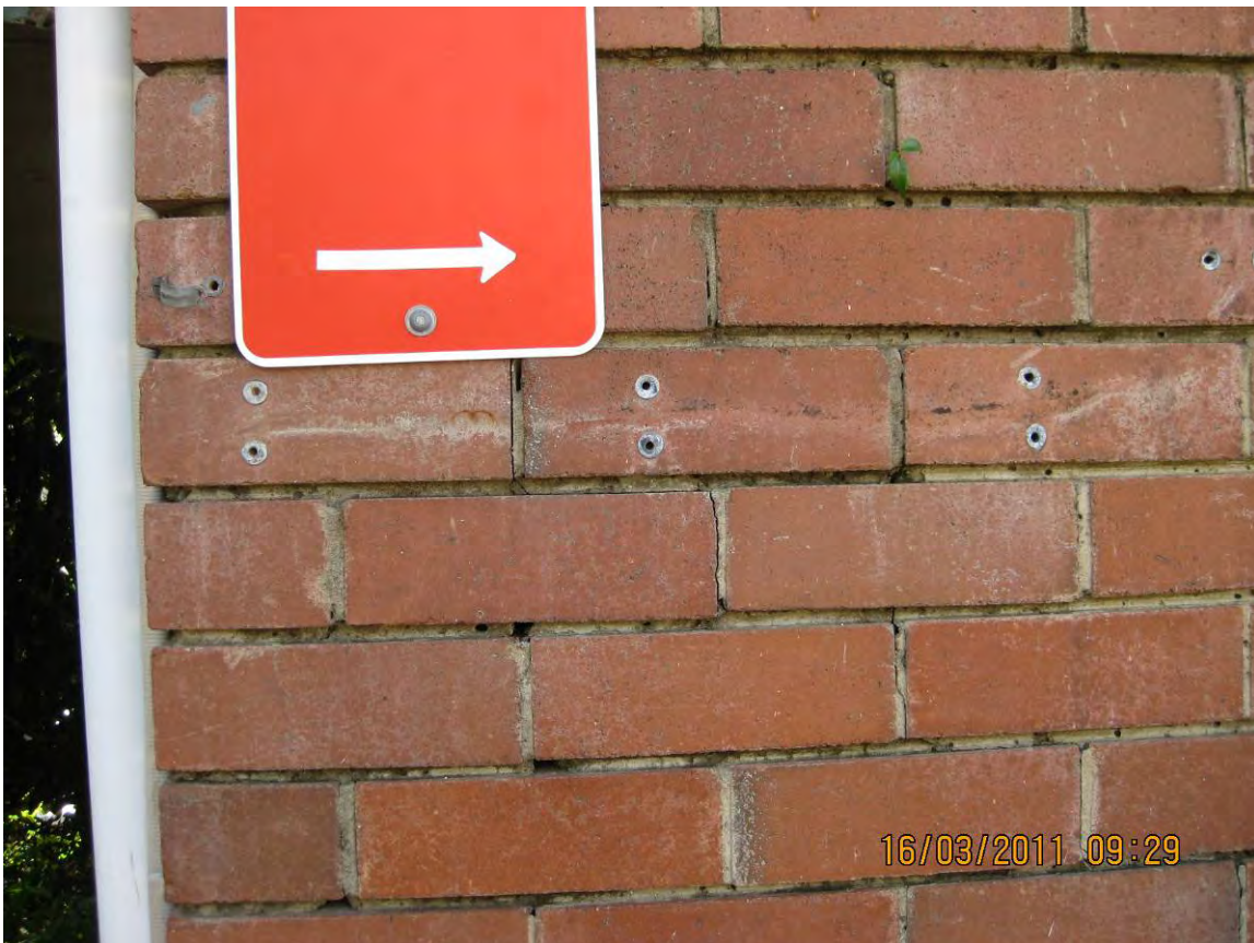
Figure 2 – Western wall crack
