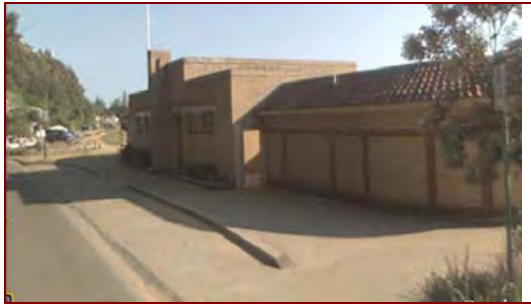
Figure 2.48: Palm Beach pavilion (Google Earth).
