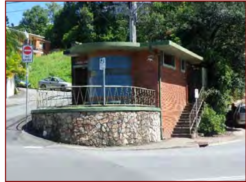
Figure 3.15: Southern elevation showing the retaining wall
