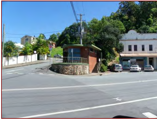
Figure 3.3: View across Queen Street to the toilet Block.
