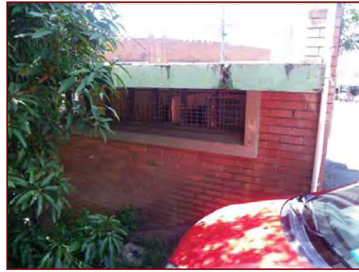
Figure 3.8: North elevation showing the rear window and roof overhang.
