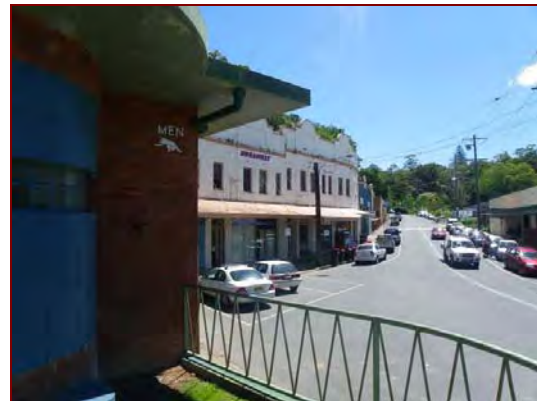
Figure 2.49: Broadway Building viewed from the Toilet Block, with the Salvation Army citadel just visible in the background.
