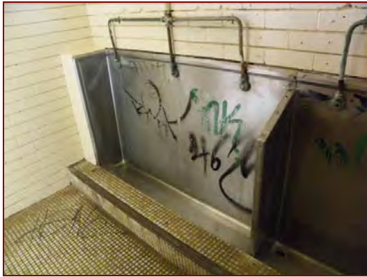
Figure 2.42: Men's urinal, note the original water spouts
