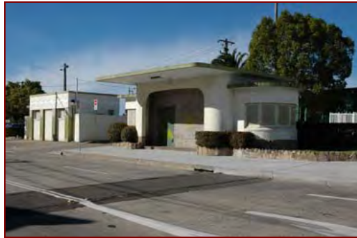
Figure 2.47: Punchbowl Bus Station, showing some similar design elements to the Toilet Block. The station is now a store room for the local park (Photo courtesy of Chris Betteridge).
