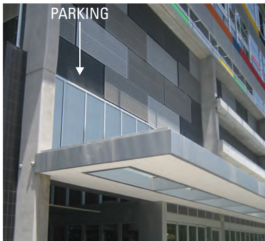
Figure 5-6: Example of above ground parking screened from public domain as a recessive element in the overall building design
