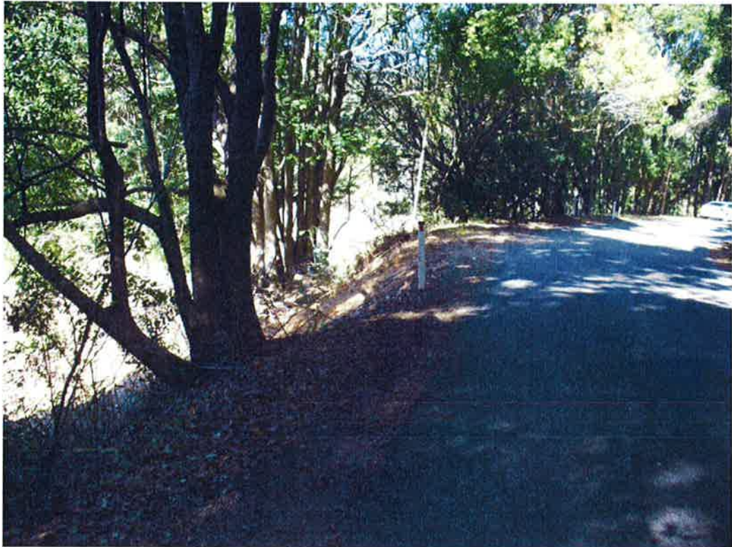
■ Figure 5-11 Steep drop off side of Cudgera Creek Road south of quarry entrance
