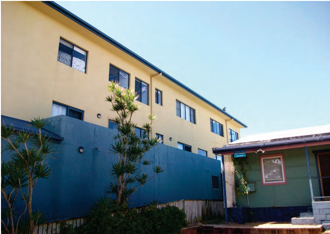
Figure 9 View of adjacent three storey units.
