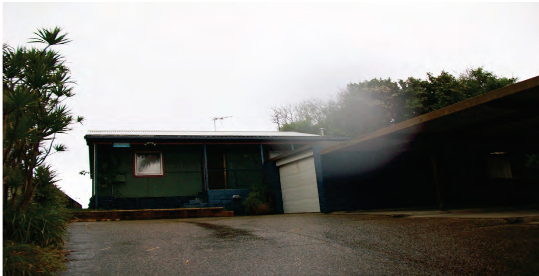
Figure 7-East view- single storey unit, garage and carport to be demolished
