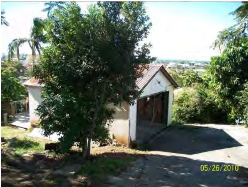
Garage associated with 13 Adelaide Street
