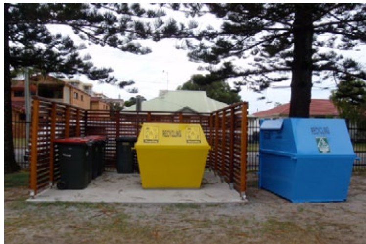
New bin Station installed at Calypso Holiday Park, Yamba.
