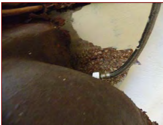
Figure 2.44: some of the original terrazzo visible behind the basin in the men's toilets.
