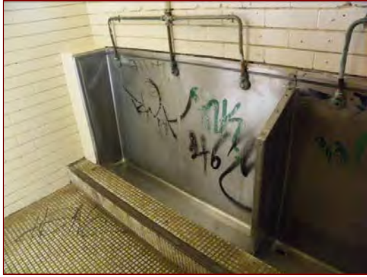
Figure 2.42: Men's urinal, note the original water spouts
