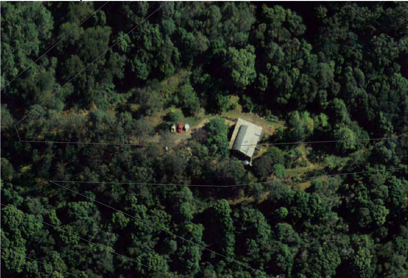
Structure in vicinity of road reserve:-
