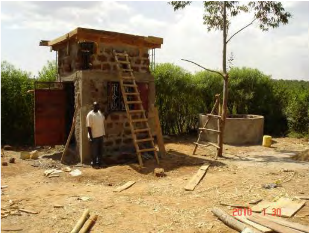
Safewater 3 kiosk under construction
