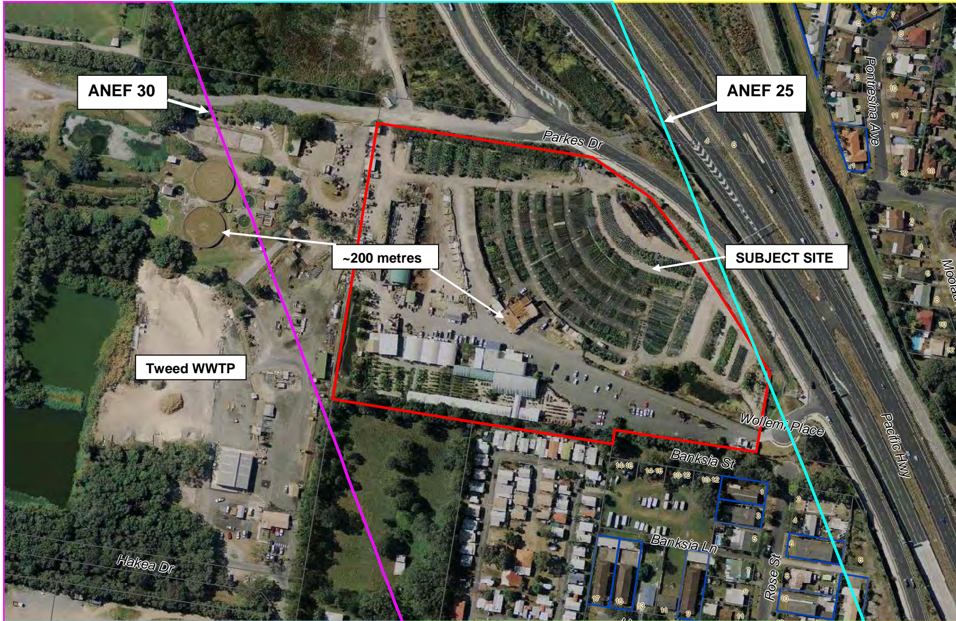
ATTACHMENT 1: Boyd's Bay Garden World Planning Proposal – ANEF 25-30 zone and indicative 200 buffer distances
