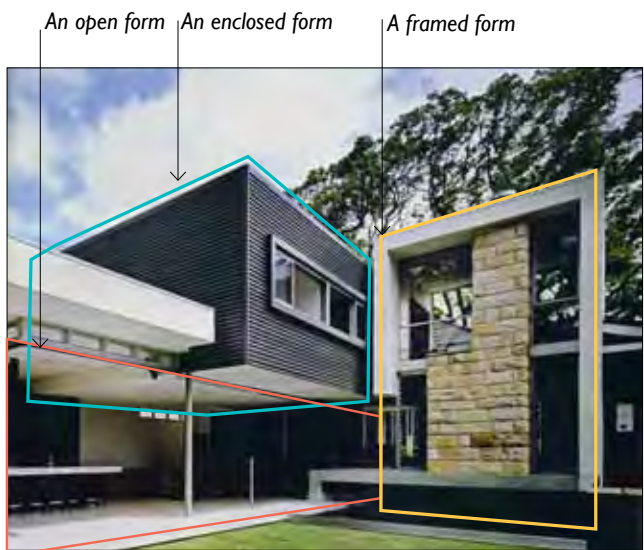
Materials are used to define forms, they wrap over and around parts of the building. Enclosed forms contrast with open frames and blade walls.
