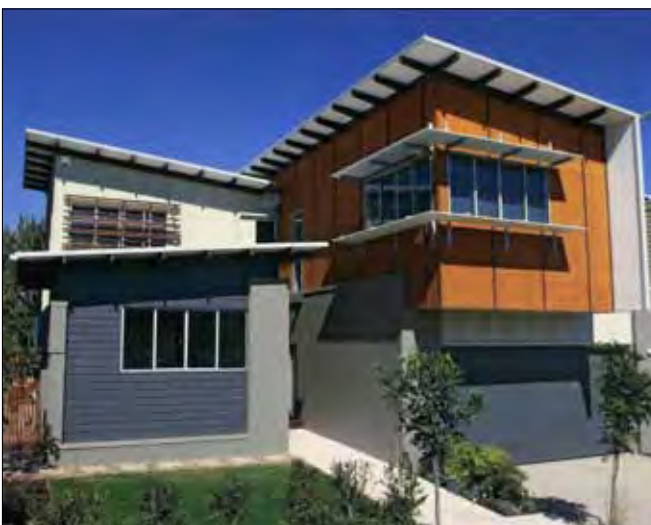
The idea of interlocking forms is expressed in this simple two storey building by the use of materials, colour and roofs.
