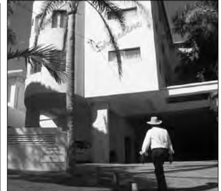
Buildings that have not concealed car access and movement areas such as ramps and carparks result in large areas of concrete and bitumen dominating the ground plane and detracting from the character of a small coastal settlement.
