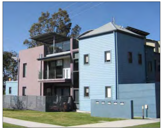
The design of this building has resulted in the appearance of a series of linked pavilions break down the bulk of the building.
