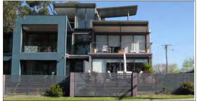
This building appears as two storeys although it is three. The third level is concealed in the roof. Fly roofs taper the building towards the sky reducing the apparent building height.
