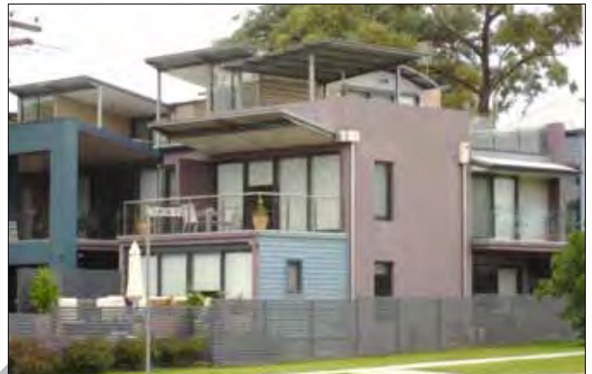
The building can be significantly reduced in height and the overall bulk of the building reduced by using a variety of smaller broken up roof forms.
