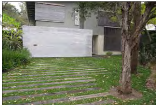
Ramps can be concealed within the buildings envelope. This avoids unsightly retaining walls, gives the building a more residential character and improves pedestrian safety and amenity on sites.
