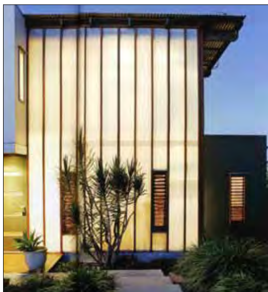
Building forms can be designed to change expression from day to night.
