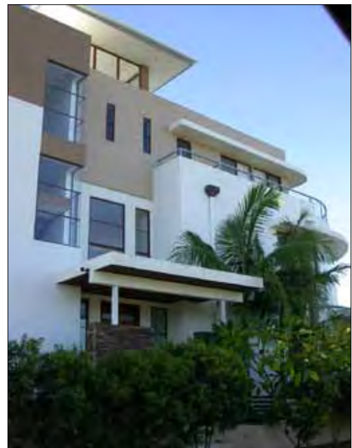
Although this building requires a greater amount of lightweight materials to be appropriate for Hastings Point and is larger than buildings will be in Hastings Point it is a good example of where the design has worked hard to break up blank walls and express the different functions and levels of the building. The variety of windows types, window shading, roof overhangs and enclosed balustrades add to a diverse elevation and break up the buildings bulk and increases internal privacy.
