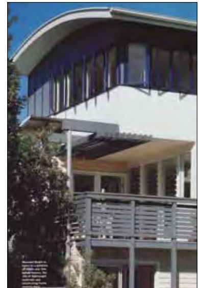
This building has a varied facade with projecting and receding areas, extended by pergolas and stepped with recessed balconies.
