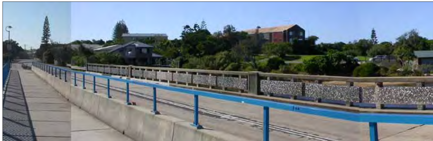
View for photomontage - From the bridge looking north
